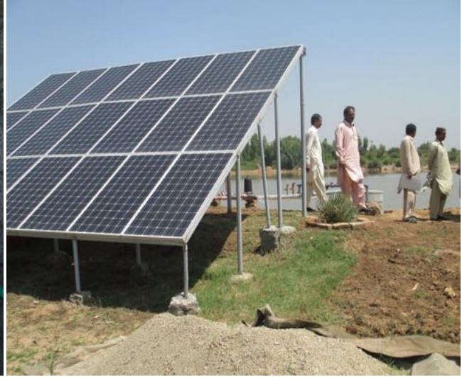
7.5 KW Solar Plant for Pump from Mini Dam
