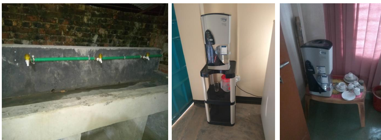
Figure 5: Drinking water facility at B # 79, Dohazari camp and Max Lab.
