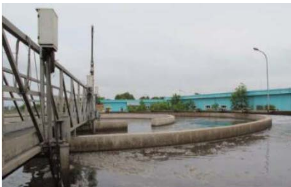
Figure 31. Wastewater treatment lagoon of Bac Giang WWTP
