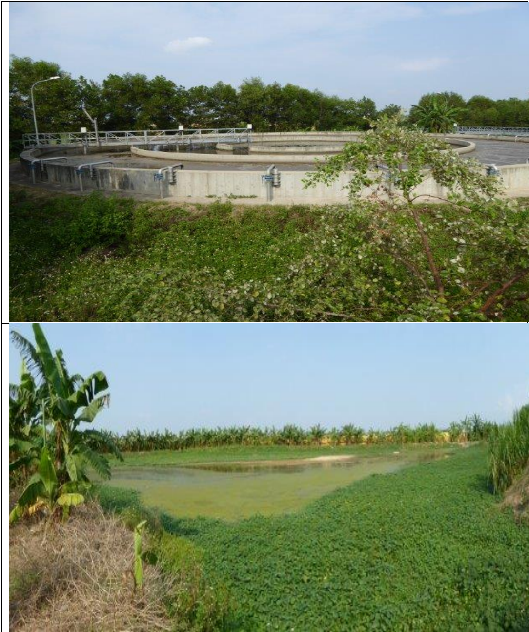
Figure 19. Existing WWTP, and planned expansion area behind facility
