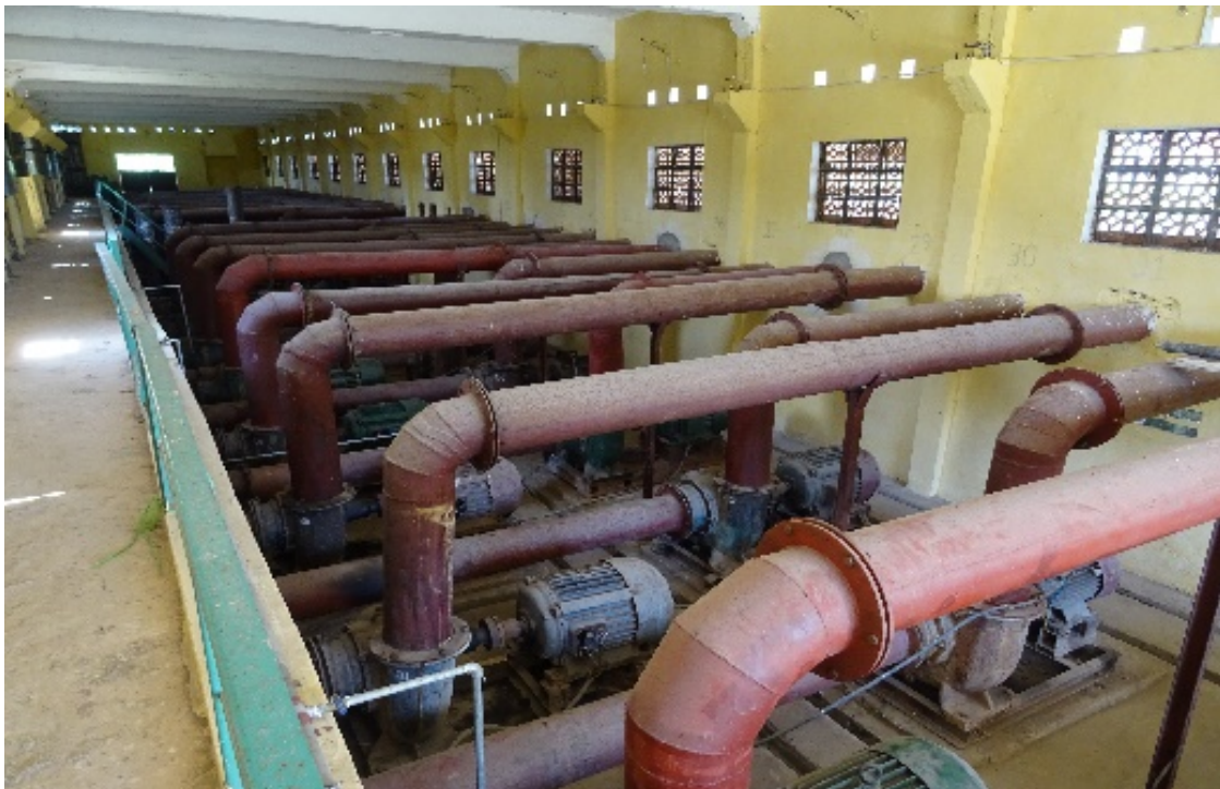
Figure 6. Existing Van Son pump station
