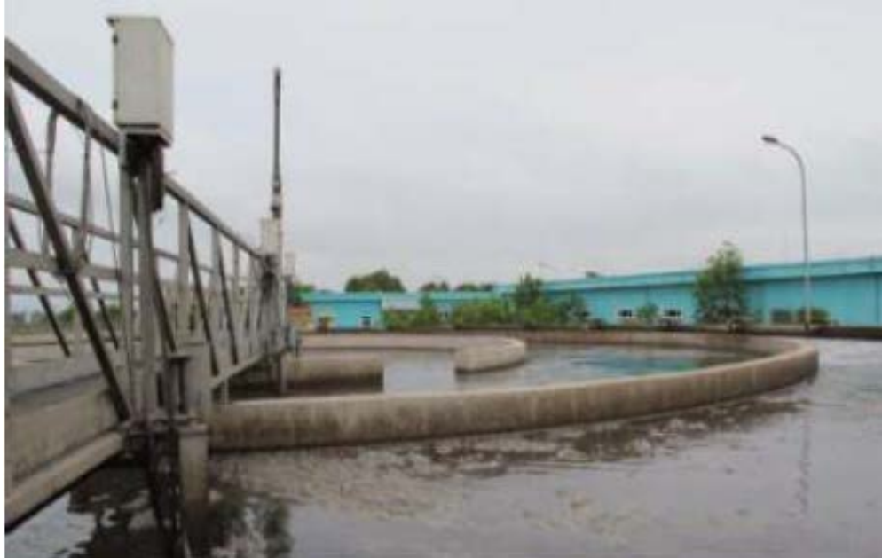
Figure 31. Wastewater treatment lagoon of Bac Giang WWTP
