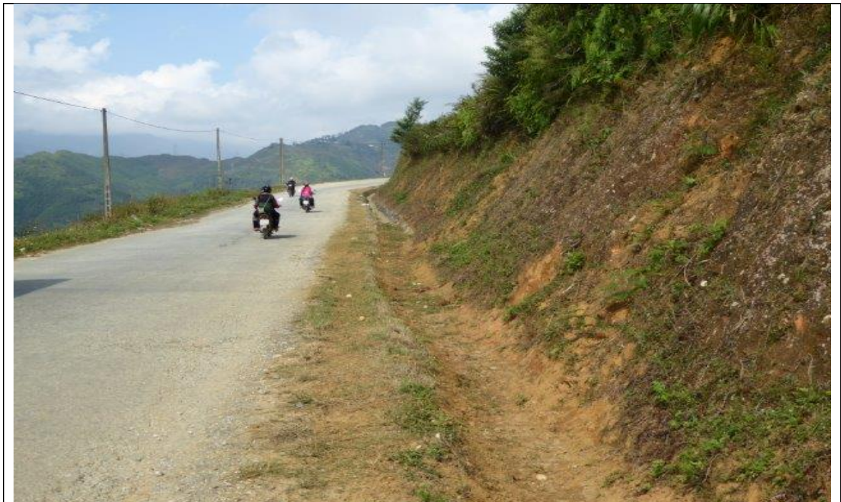
Figure 26. Sections of Road 152 southeast of Sa Pa.
