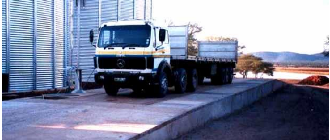
Figure 13 Typical Weigh Bridge (Flat Bunker)
