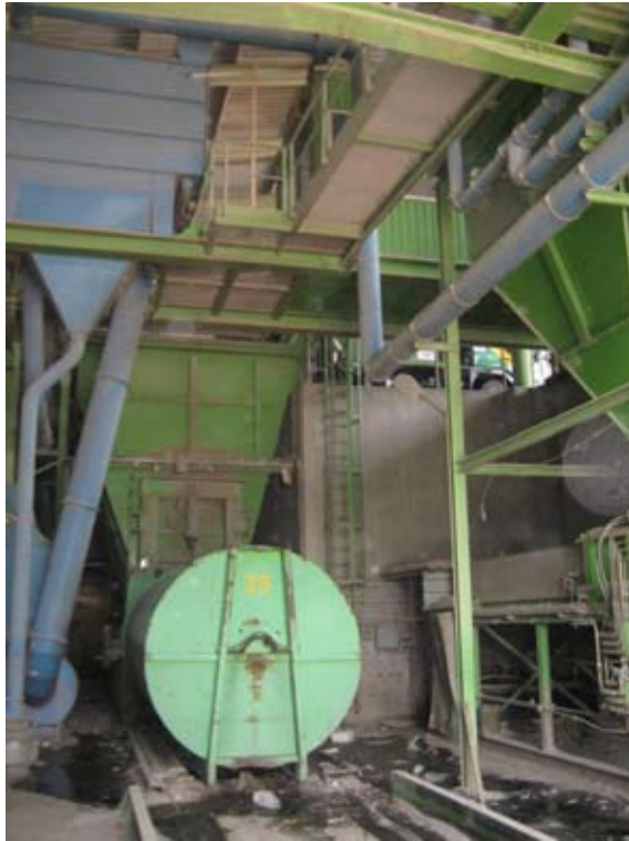
Installed Push Press System
