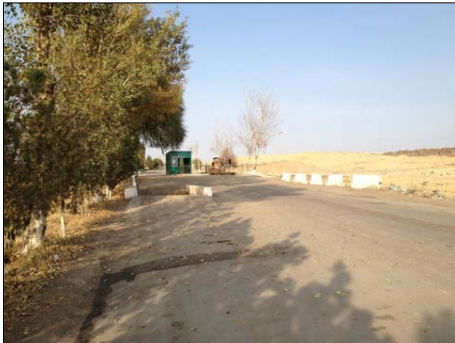
Picture 3 Weigh Bridge Area – Akhangaran Landfill
