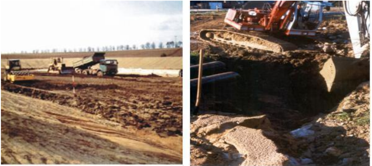
Picture 7 Earthmoving activities during site preparation for the Establishment of a landfill
