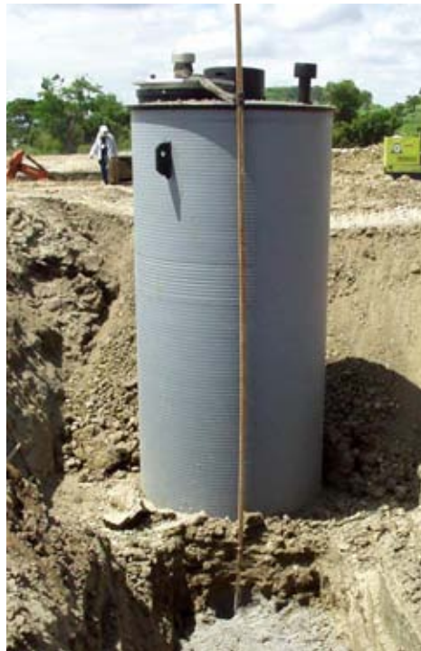
Figure 12 Leachate Collection Shaft
