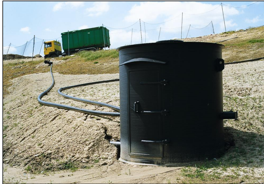
Picture 11 LFG well head and LFG collection station
