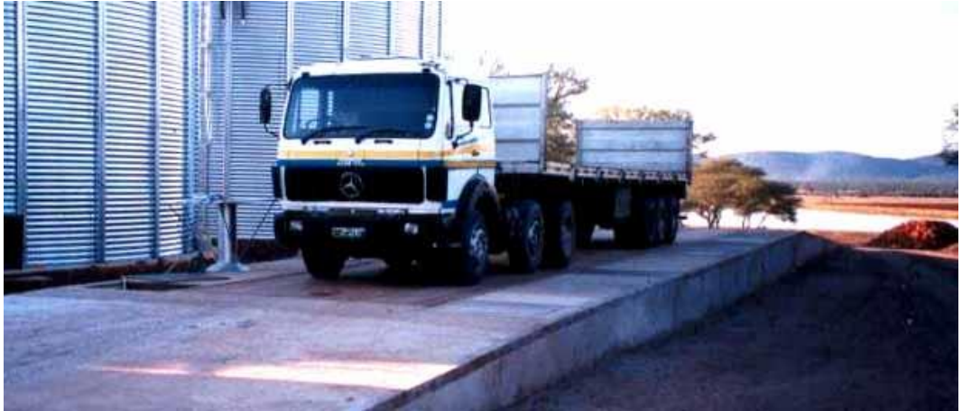
Figure 13 Typical Weigh Bridge (Flat Bunker)
