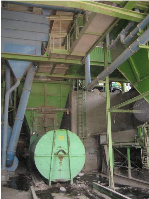
Installed Push Press System
