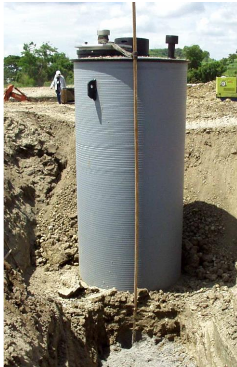
Figure 12 Leachate Collection Shaft
