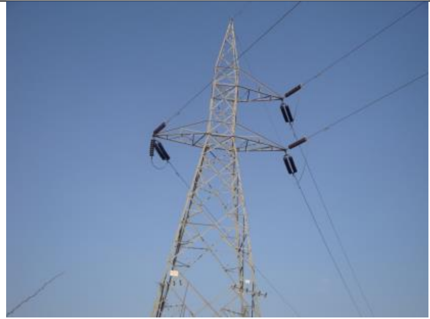
Figure 3.23 B: LIL tower at Jaatipura
