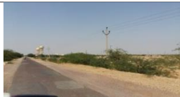
Existing water pumping state in buffer area
