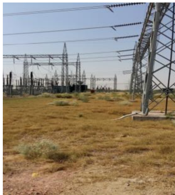
Figure 3.18 Land for bay for 220 kV Chhattargarh – Gajner at Gajner
