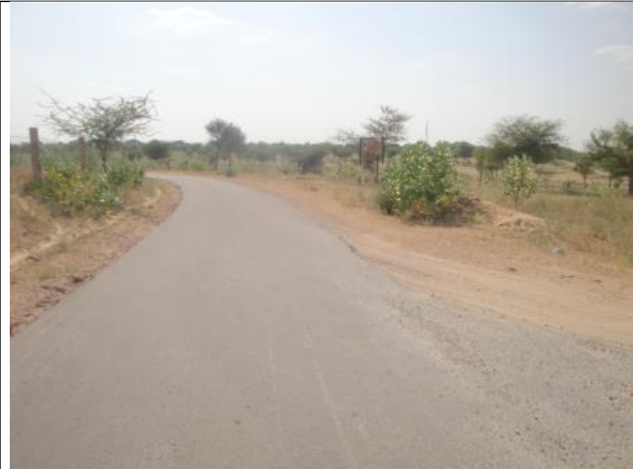
Figure 3.21B: 132 kV Dechu Nathrau line road crossing
