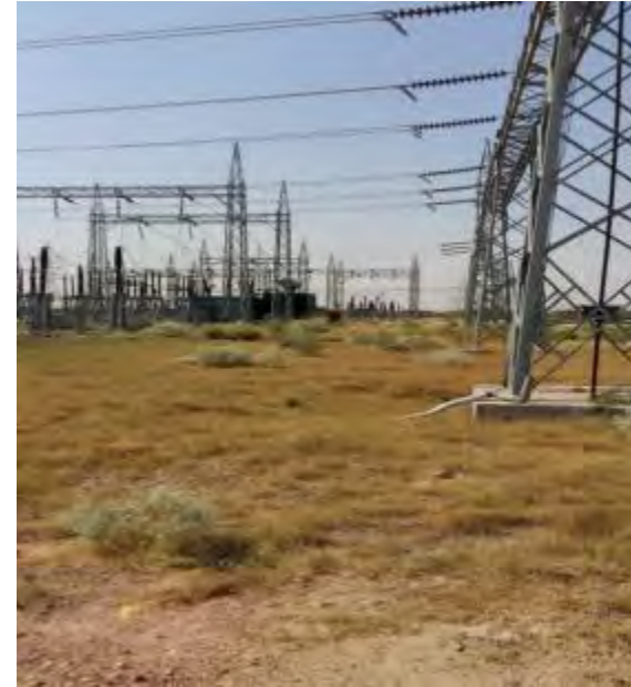
Figure 1.18 Land for bay for 220 kV Chhattargarh – Gajner at Gajner
