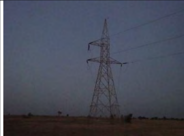
Figure 1.22B: 132 kV LILO line to Sangarh GSS
