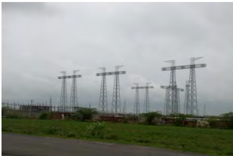
Figure 1.7: Photograph of 765 Ajmer GSS (Powergrid)
