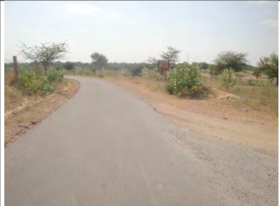
Figure 1.21B: 132 kV Dechu Nathrau line road crossing
