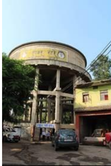
OHT at Shanwara Ward at Burhanpur
