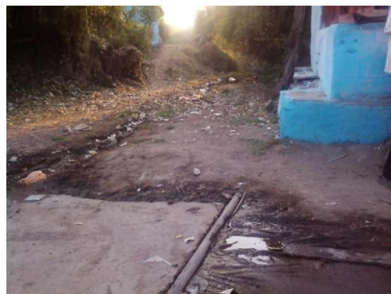
Absence of Sewerage System
