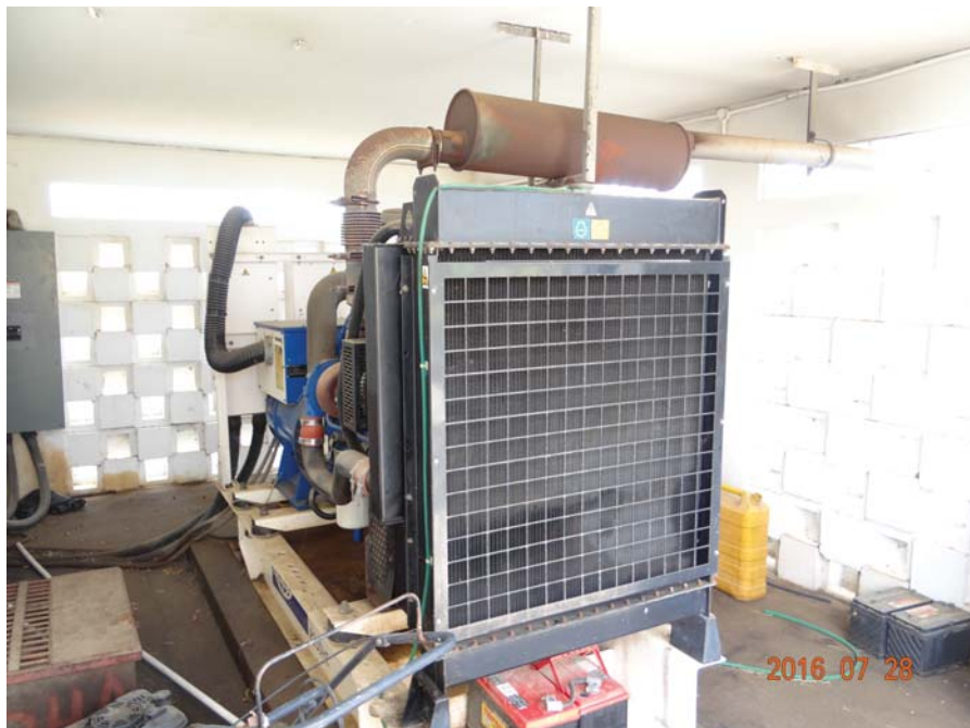
f) Back-up generator
