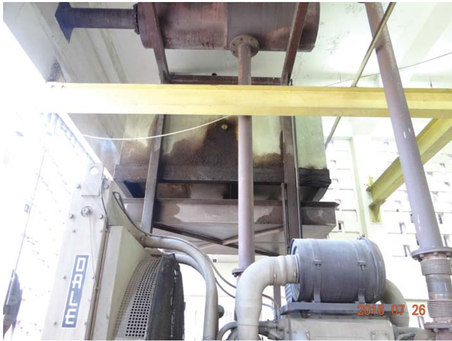
d) Back-up Generator
