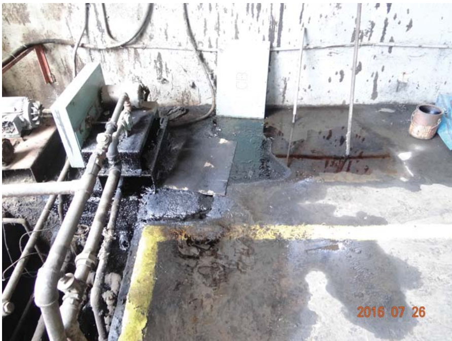
c) Boiler room floor (oil spill)
