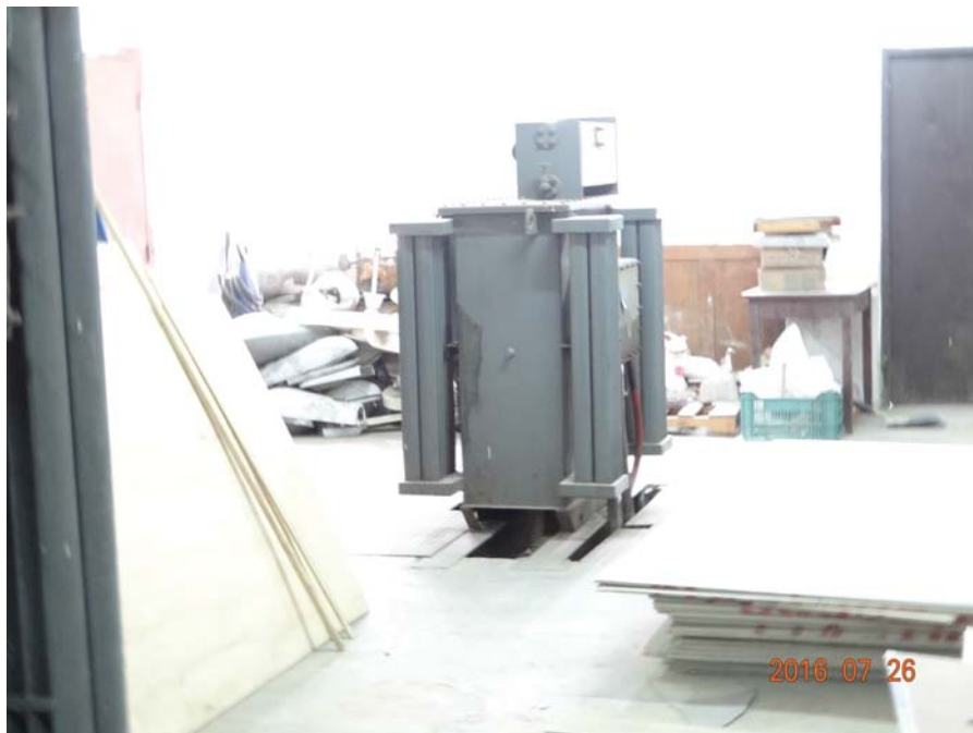
f) Leaking transformer
