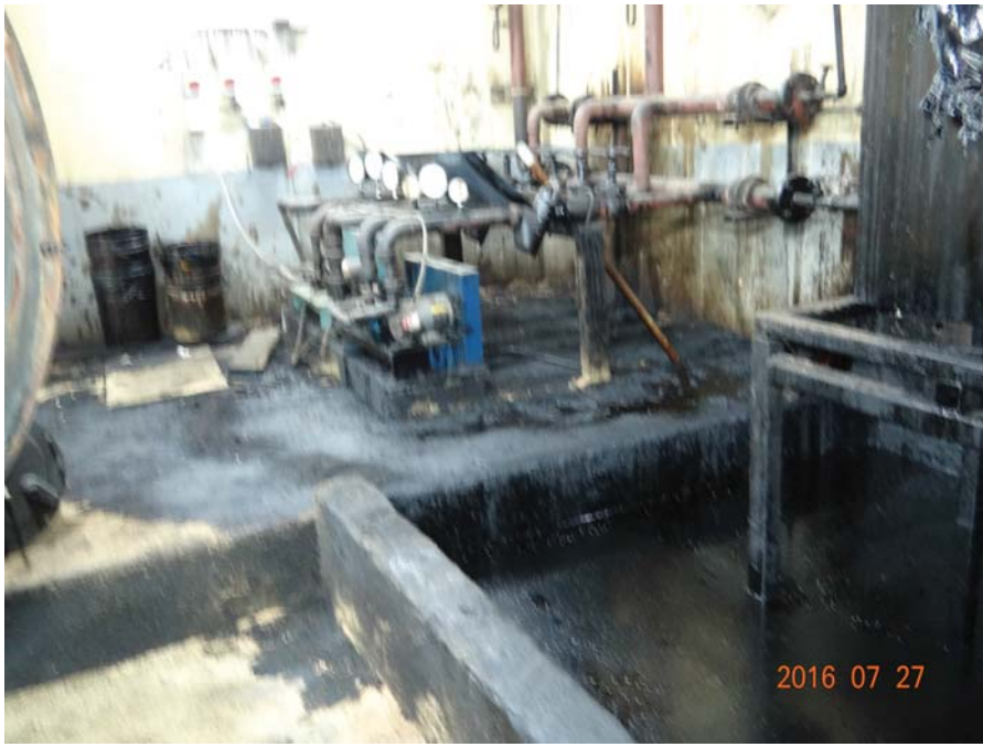
d) Boiler room and spill
