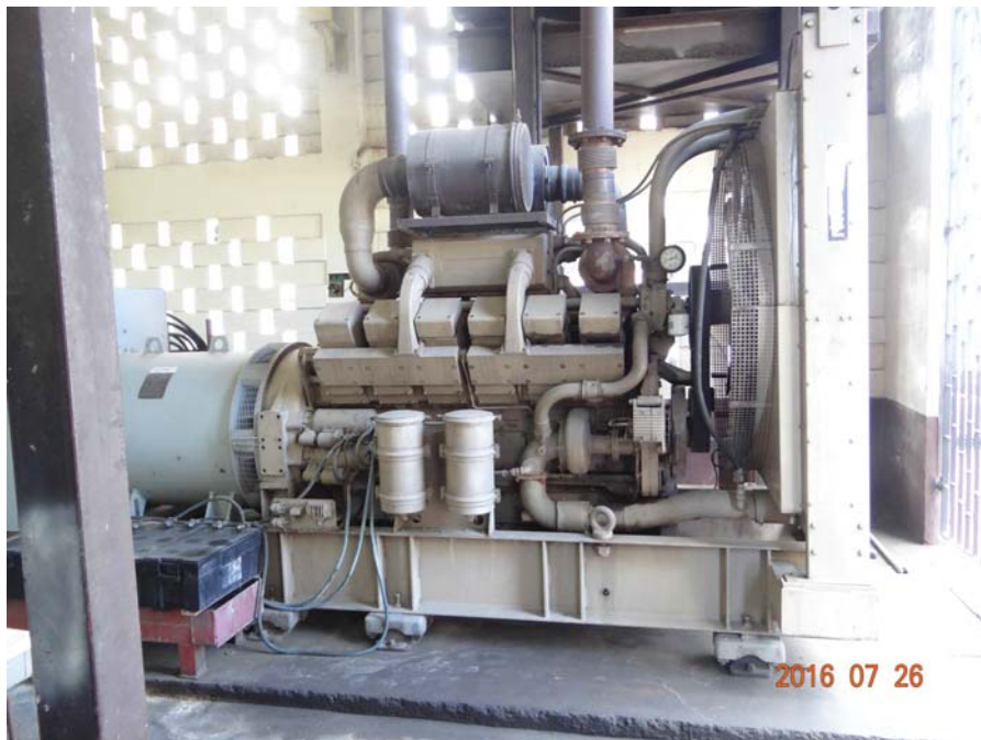
e) Back-up Generator
