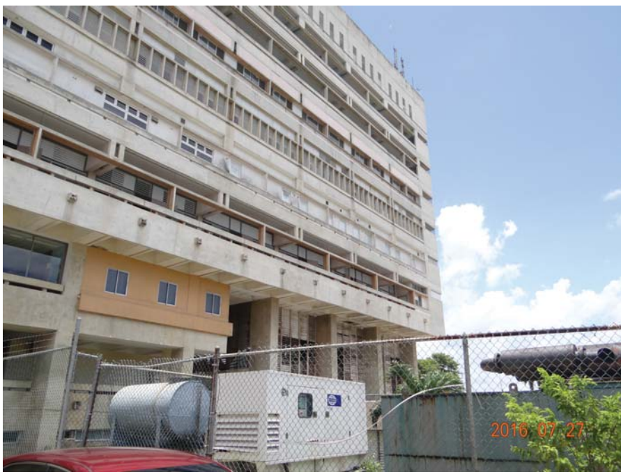
e) Windows, back-up generator and fuel tank
