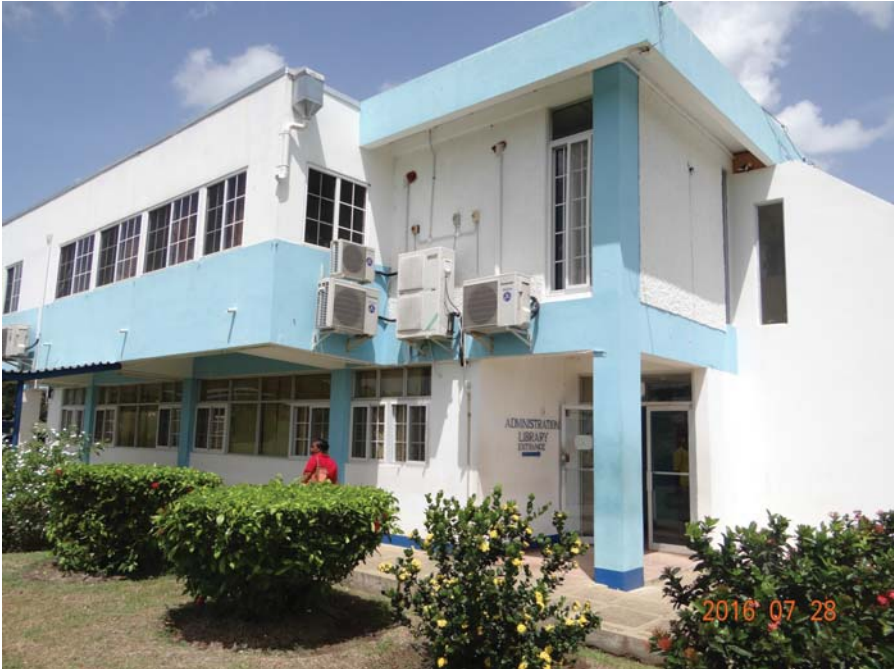
b) General view (incl. coolers and open windows)
