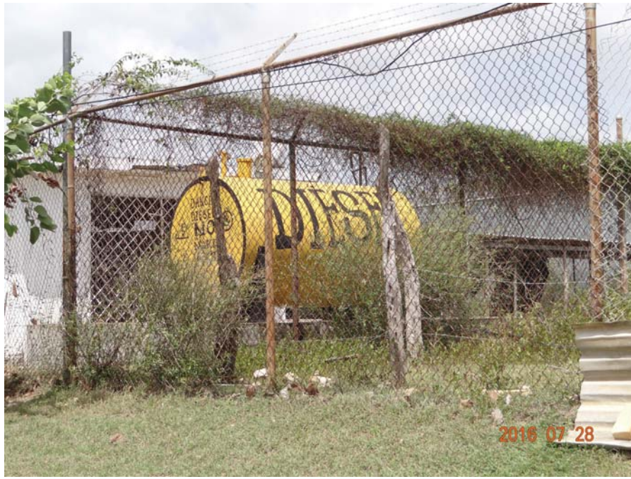
d) Storage tank for back-up generator
