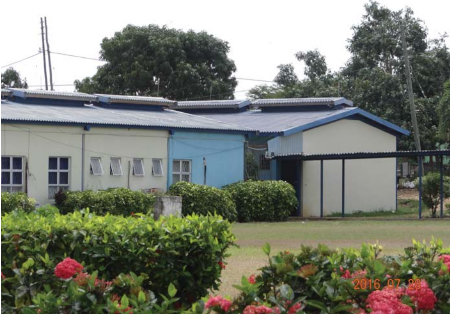
c) Classroom / lab, (corrugated roofing, and open windows)
