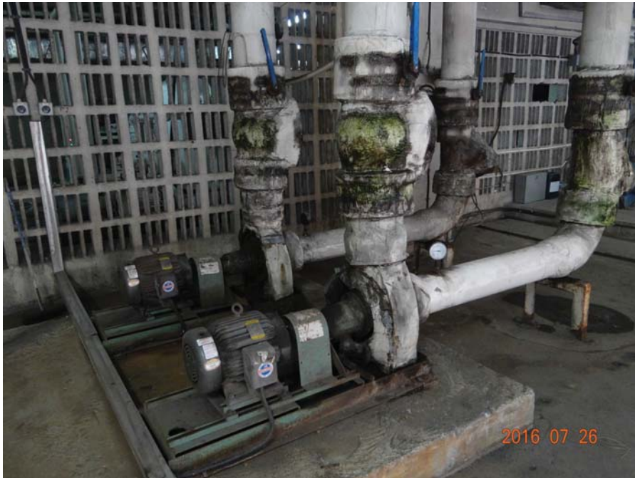
h) Main water pumps
