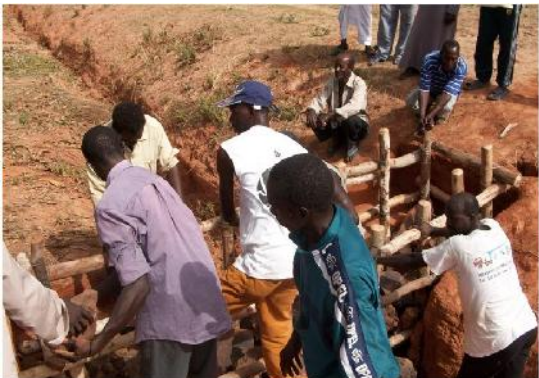
Fig. 7: Construction of a frame bund
