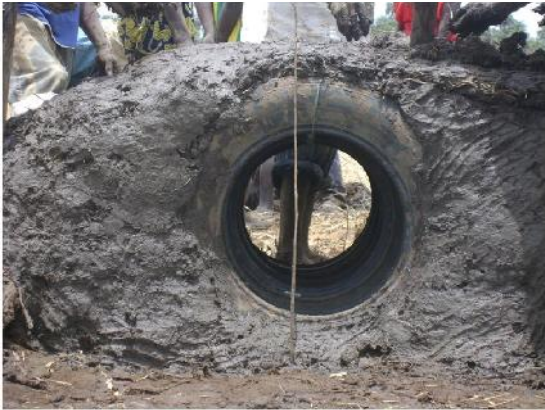
Fig 6: Use of used tyres to build an outlet
