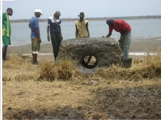
Fig 6: Use of used tyres to build an outlet
