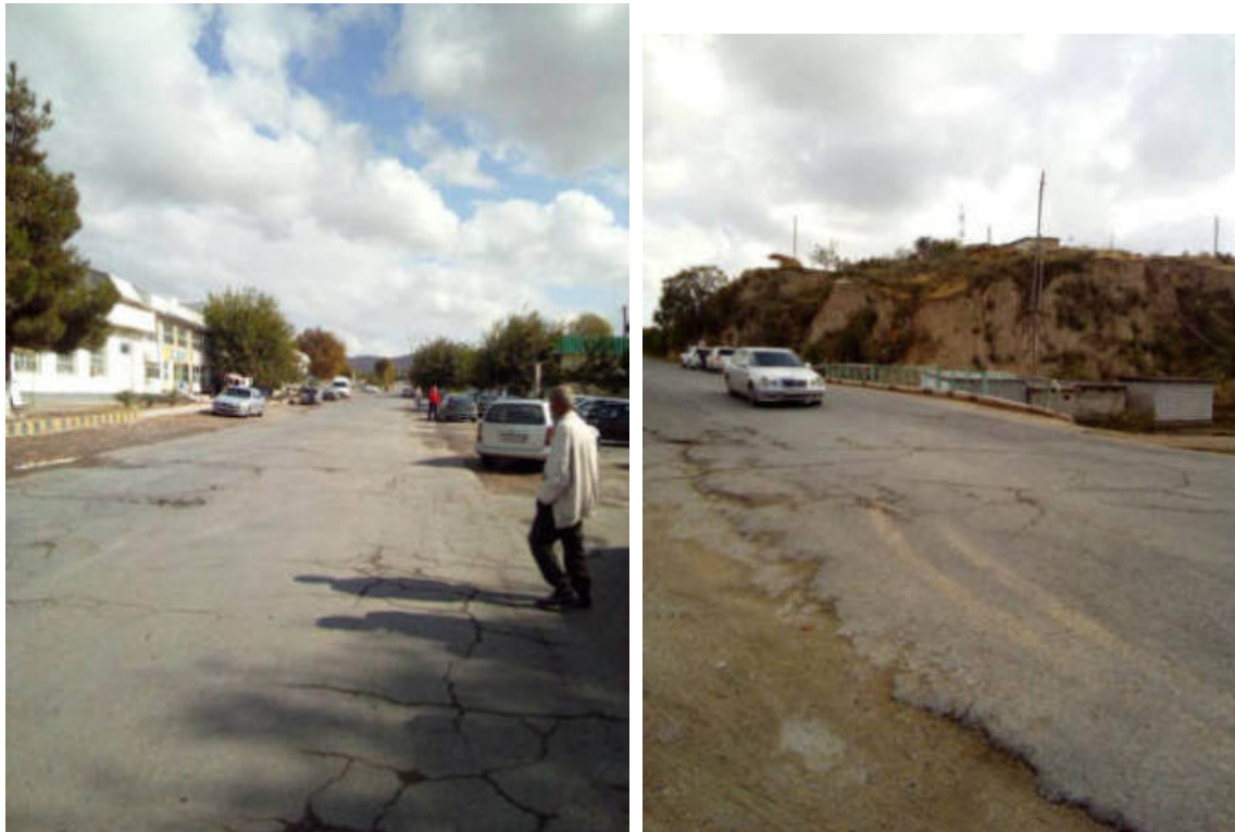
Figure 6 - Severely Damaged Road Pavement
