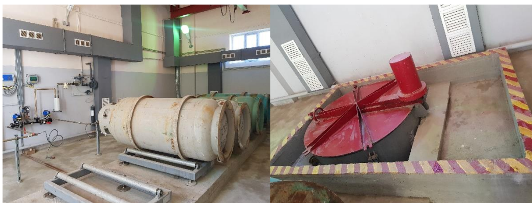
Figure 5 Chlorine tanks and sarcophagus
