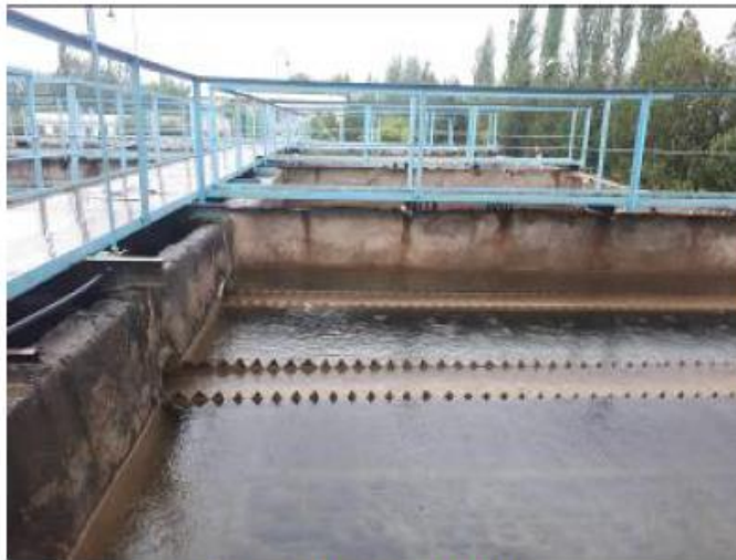
Treatment line for 50,000 m 3 /day
