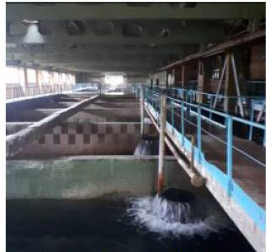
Treatment line for 80,000 m 3 /day
