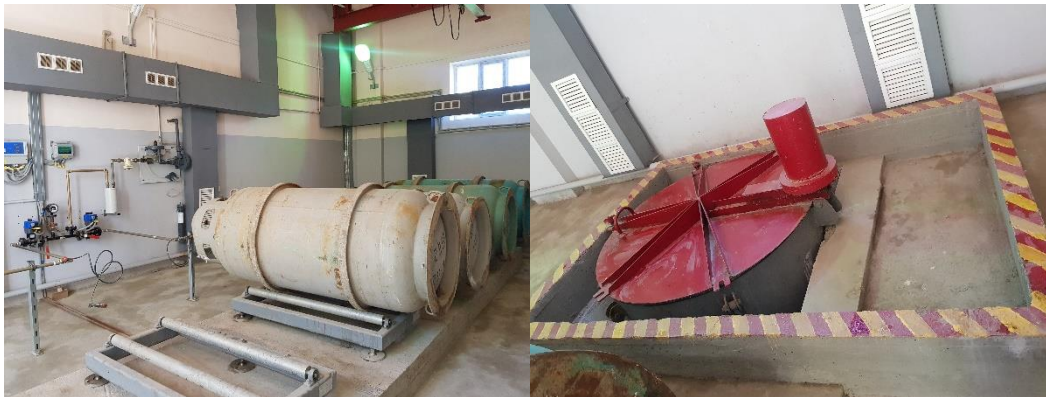
Figure 5 Chlorine tanks and sarcophagus
