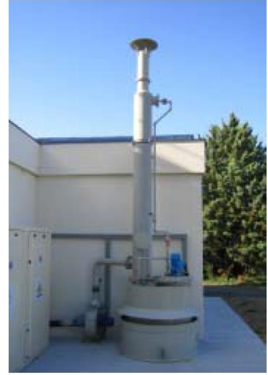
Figure 8 Examples of Chlorine Neutralization Facilities
