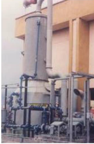
Figure 8 Examples of Chlorine Neutralization Facilities
