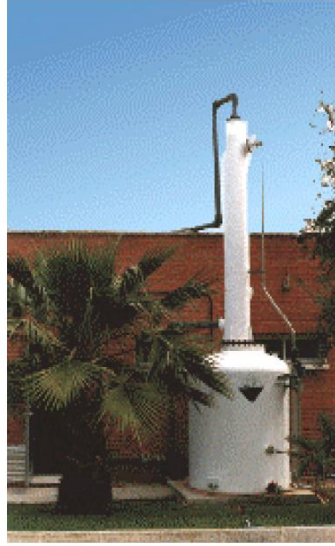
Figure 8 Examples of Chlorine Neutralization Facilities
