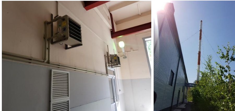
Figure 6 Ventilation system and stack
