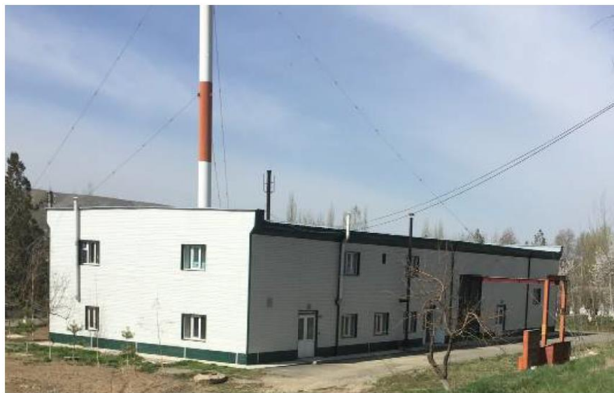
Figure 3 Chlorination Plant in Ozgor WTP
