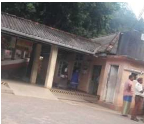
Asbestos roofing sheets & ceiling sheets to be removed during demolition at Welmada BH
