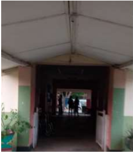
Asbestos roofing sheets & ceiling sheets at Medirigiriya BH
