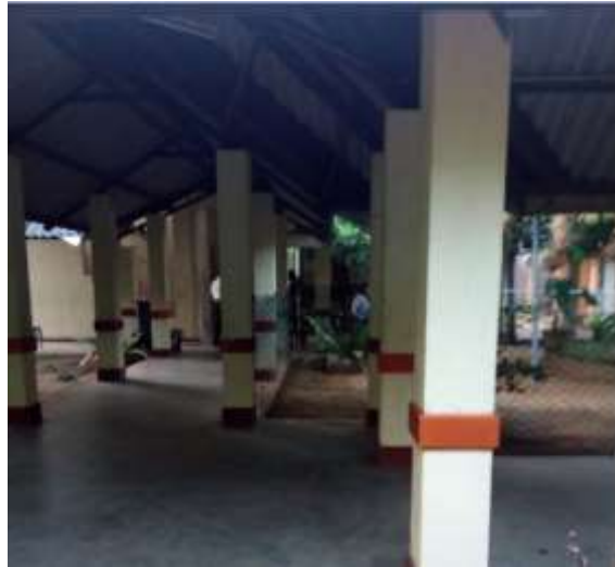
Asbestos roofing sheets & ceiling sheets at Medirigiriya BH
