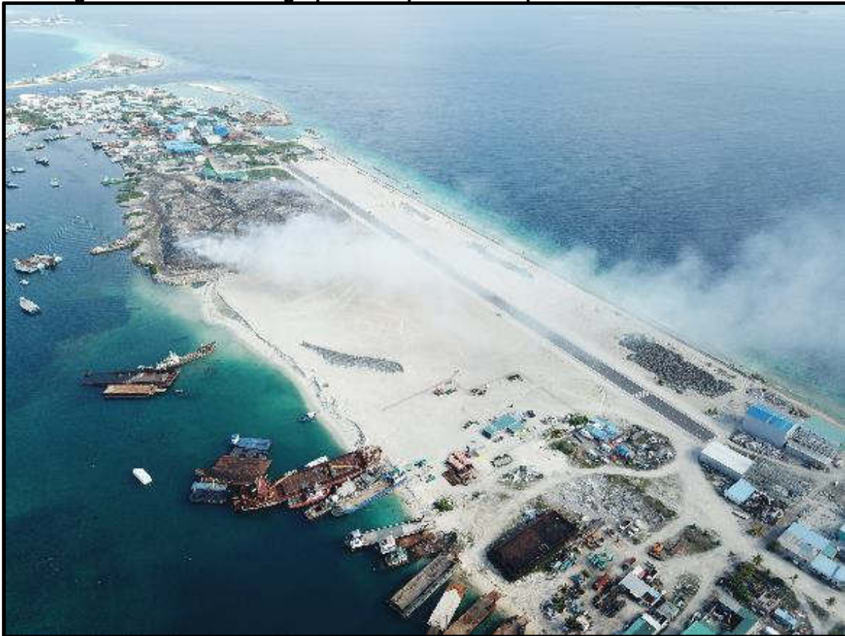
Figure 61: Aerial Photograph of Proposed WTE plant Location at Thilafushi
