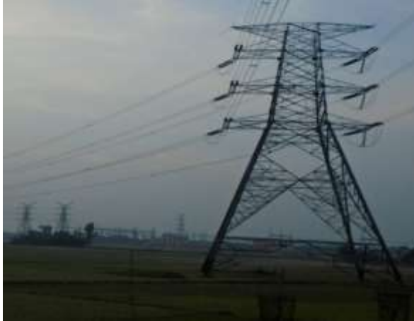
Photograph 1.1: Tension Tower (230 kV TL)
