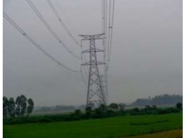
Photograph 1.2: Suspension Tower (230 kV TL)
