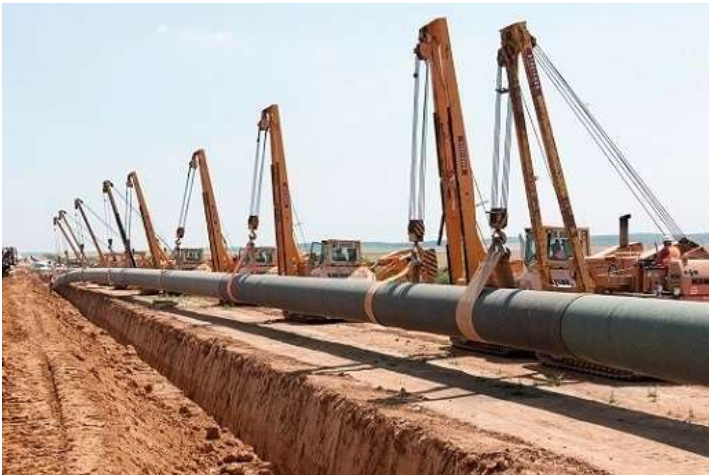
Photograph 1.1: General View of Gas Pipeline Laying
