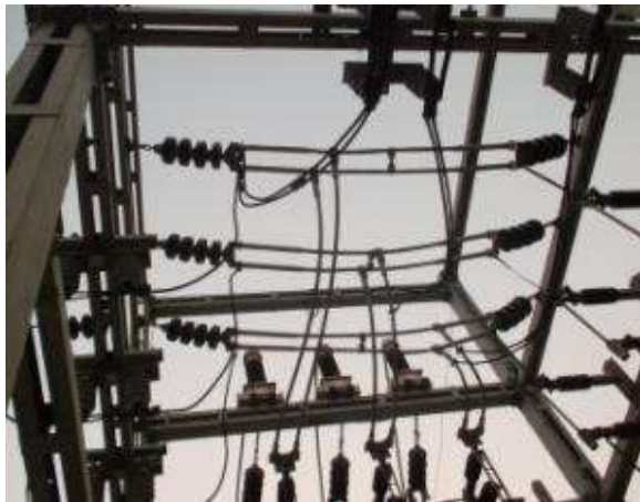
Photograph 1.3: Disc Insulators for transmission line
