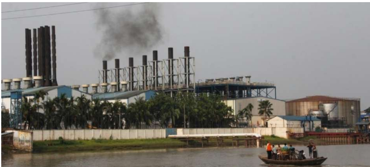
Existing power plant by the Bhairab River, 31 May 2017.
