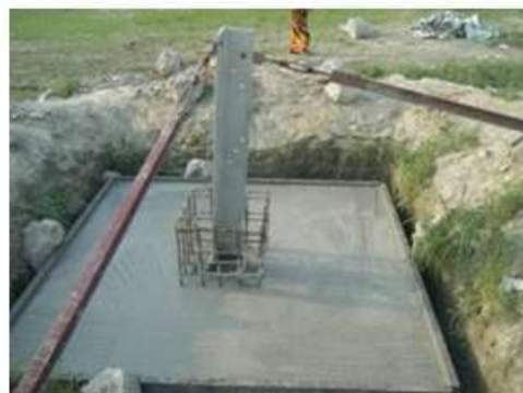
Casting CC into tower foundation
