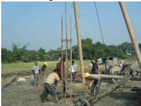
placing of steel ring bunds
