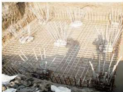
pile cap reinforcement
