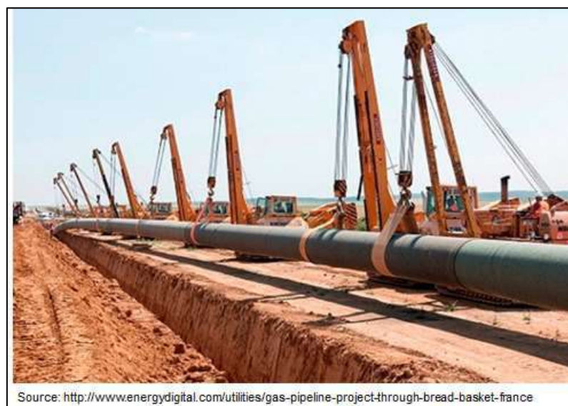
Figure 3.8: Laying of Pipeline
