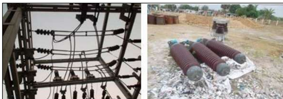
Figure 3.3: Disc insulators for transmission line
