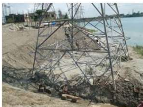
Placing tower on its foundation
