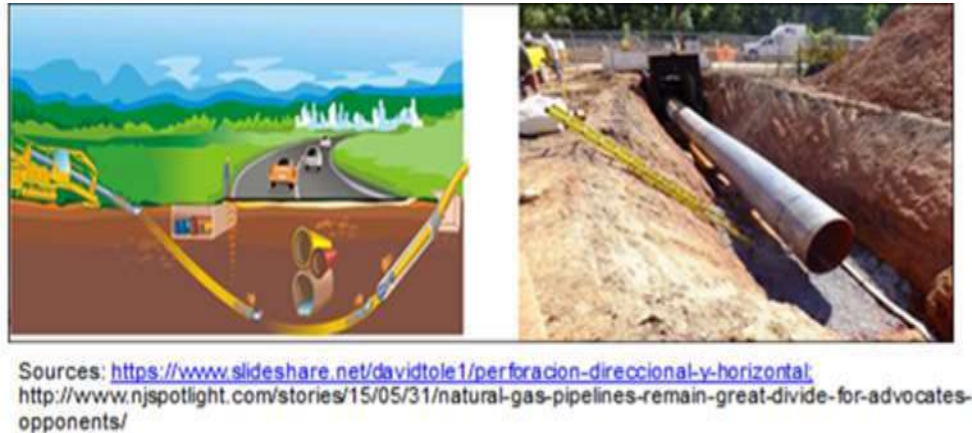
Figure 3.7: HDD process
