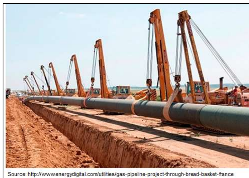
Figure 3.8: Laying of Pipeline
