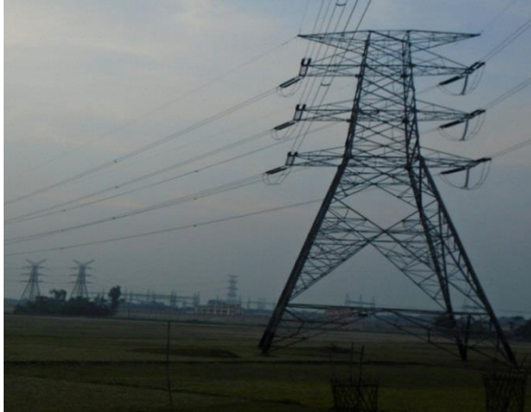
Photograph 1.1: Tension Tower (230 kV TL)
