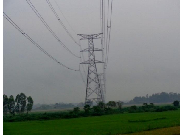
Photograph 1.2: Suspension Tower (230 kV TL)
