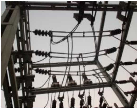
Photograph 1.3: Disc Insulators for transmission line
