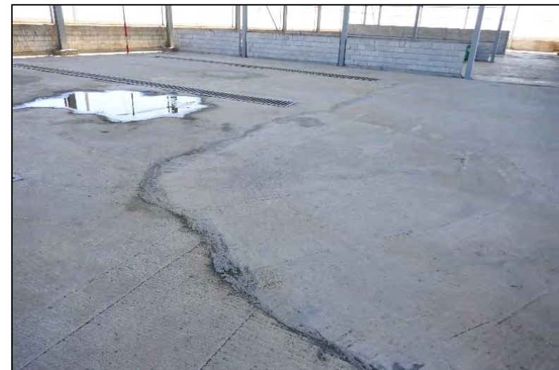
Interior of the main hazardous waste storage area
