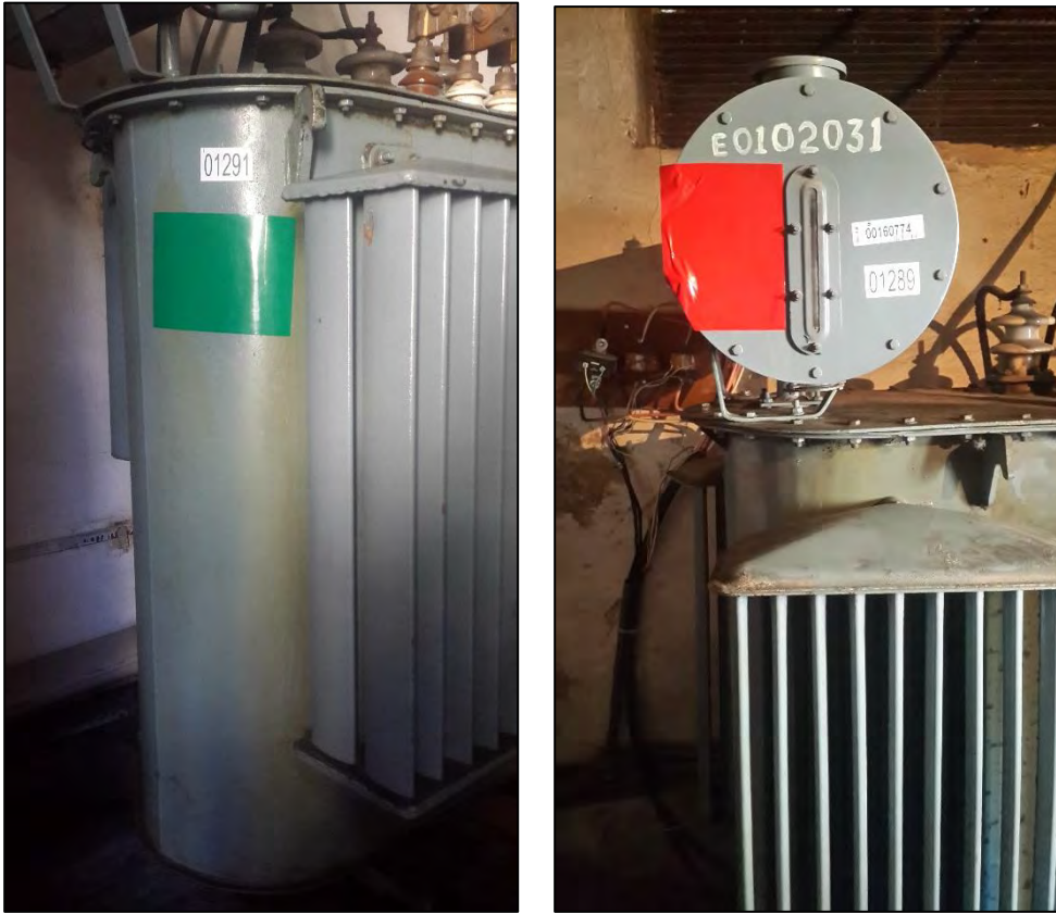
Figure 11. Labelling of Equipment with Potential PCBs
