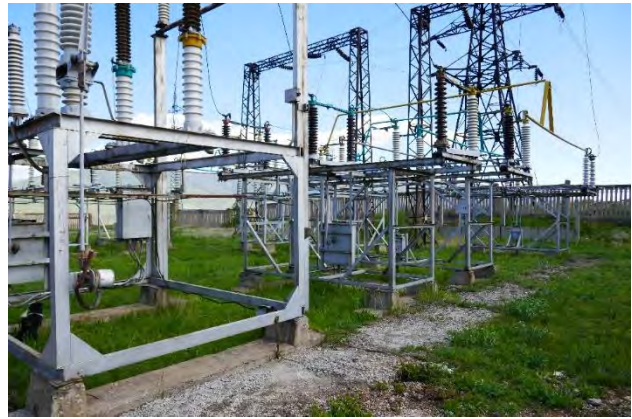
Equipment to be replaced under Phase 2 at Charentsvan City substation (110 kV, 35 kV, 10 kV)
