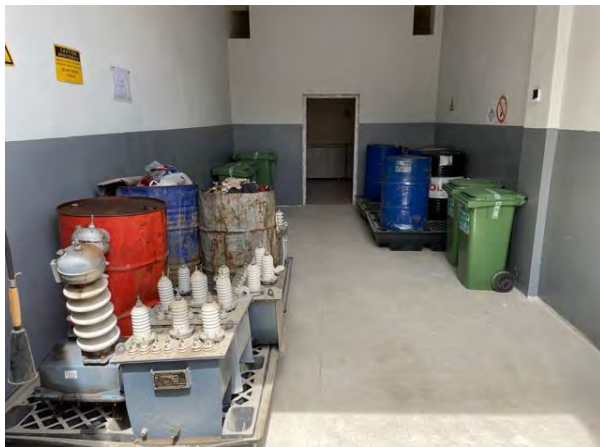
Temporary hazardous waste storage area
