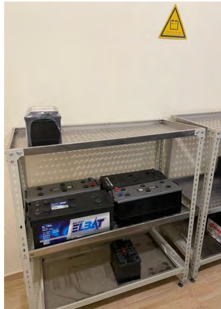
Used battery storage area
