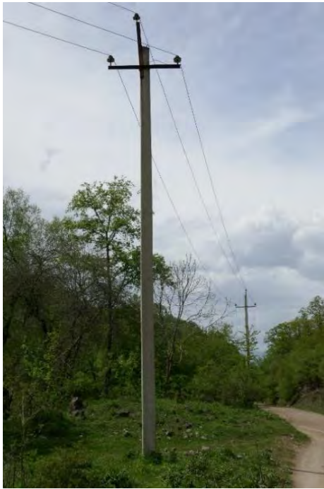
New 10 kV line near the village of Lorut
