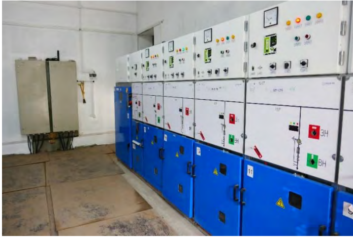
Interior of newly constructed substation in Shengavit District, Yerevan
