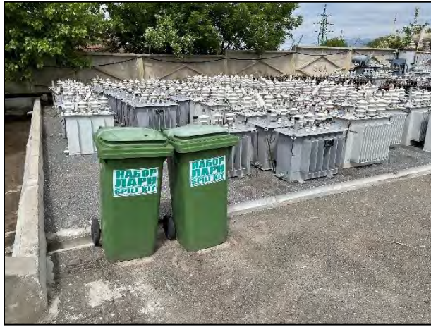
Oil spill containment area for transformers
