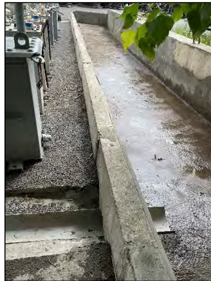
Oil containment reservoir
