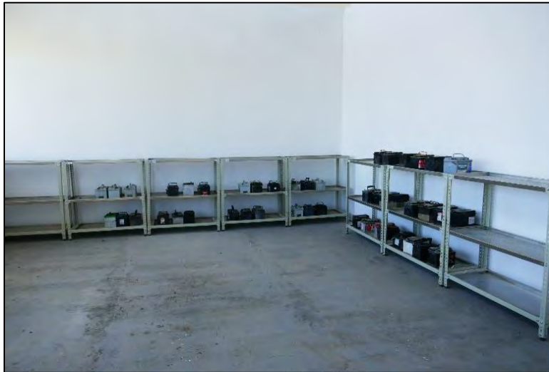
Used battery storage area
