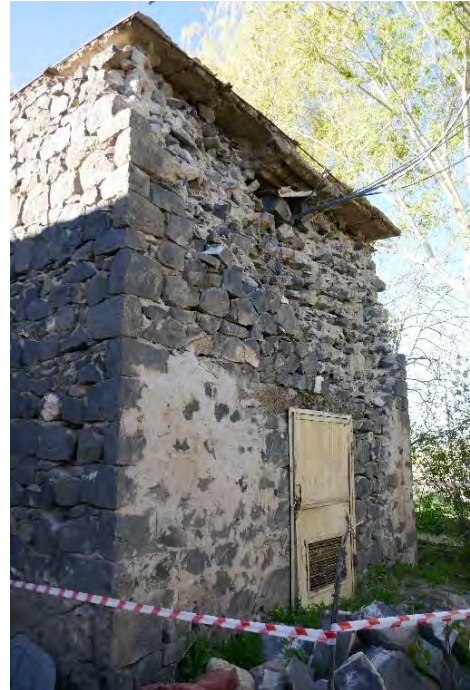
Damaged substation housing to be removed and replaced in Vardenik
