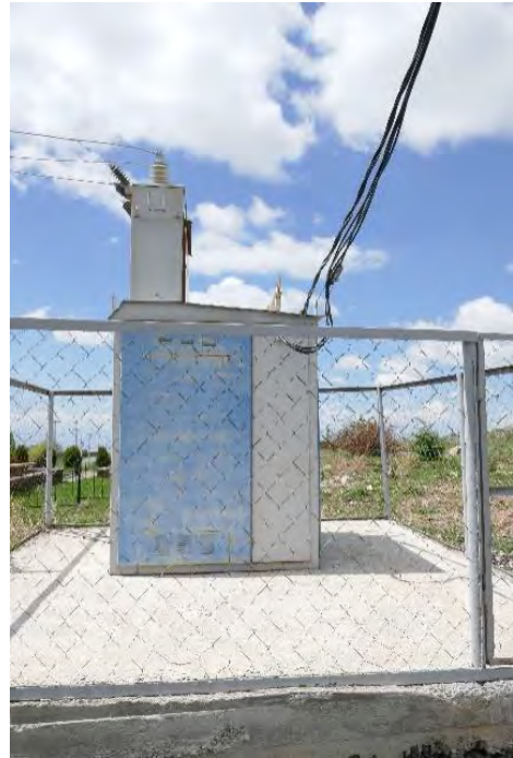
New 10 kV – 0.4 kV kiosk transformer in Avan Village
