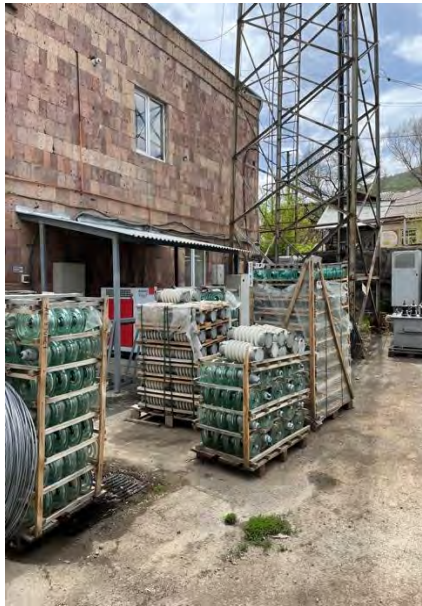
Material and equipment staging area
