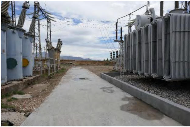
New walkways and oil containment system at Ararat Power Electric Power Substation – 1
