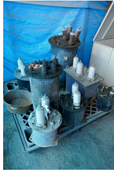
Oil containing equipment on leak containment pallets
