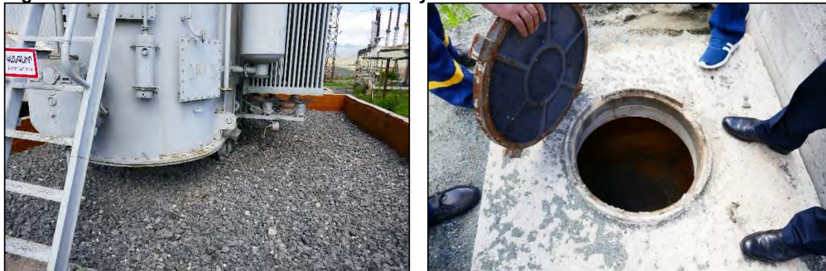
Oil containment system for transformer
