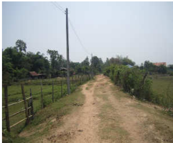
Access road to SWTP in Phonexay village.
