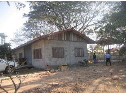
The hospital storage area on the northwest of the site.
