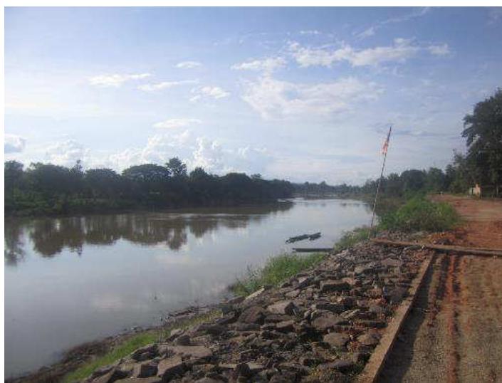
Figure 22: Unprotected bank of San River
