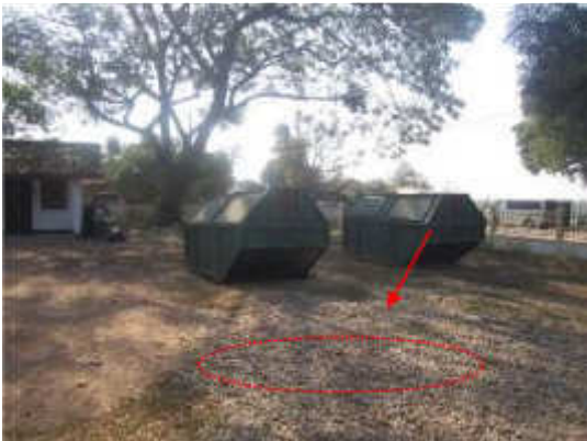
Location of SWTP at Borikhamxay Hospital Compound
