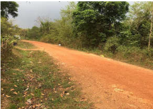
Laterite road, approximately 1 km long to the landfill site. The road passes through the Nasommo village.
