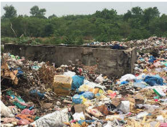
The damaged leachate collection/treatment tank.
