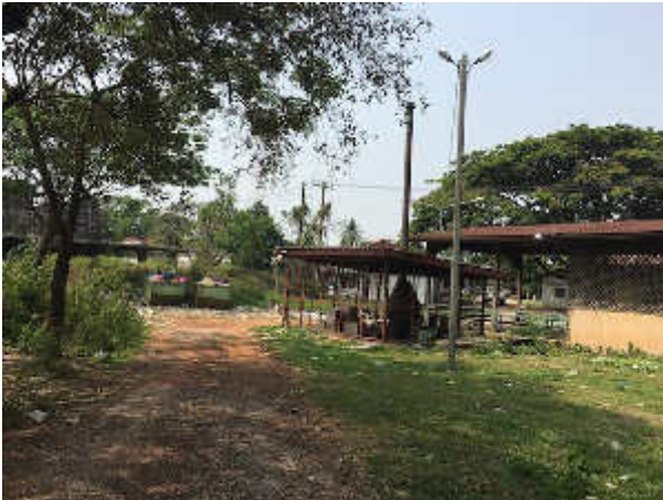
Location of SWTP at Khammoune Provincial Hospital Compound near the waste storage building and incinerator.
