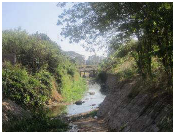
The receiving Houay Sakham of SWTP leading to Mekong River.
