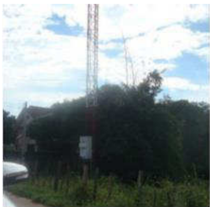
Cell tower within Drain 5
