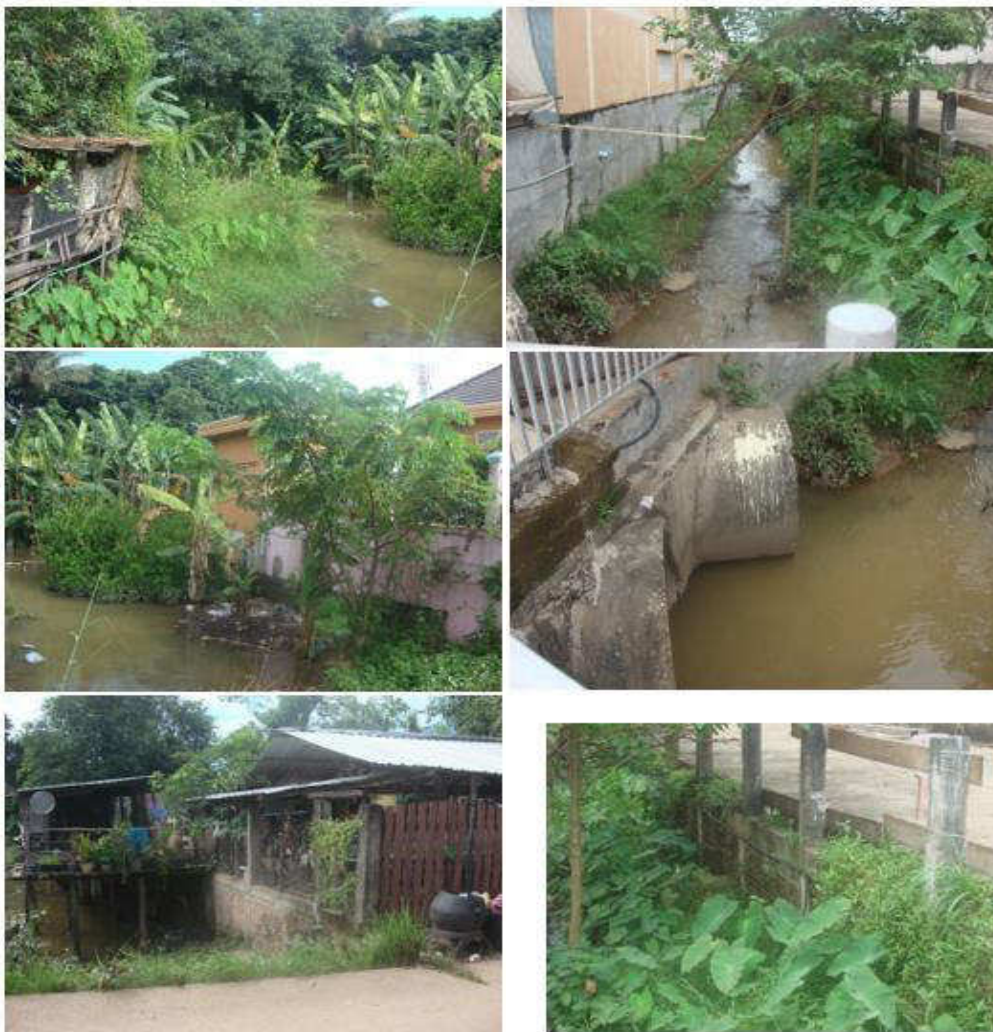
Drain 4 Drain 5 Structures immediately adjacent or encroaching and water pipes within natural drainage courses
