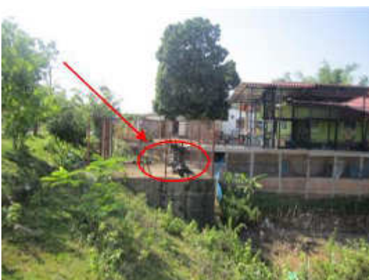
The existing floodgate at Houay Nam Sot.
