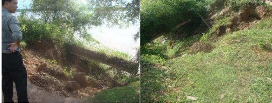
Line D: Riverbank protection from south at That Sikhottabong to north (1770m)
