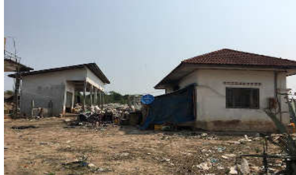
Guardhouse/office and waste weighing and baling area
