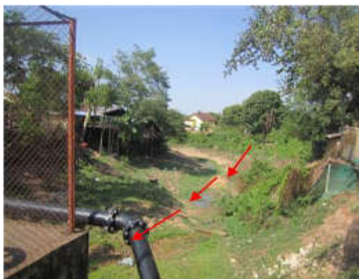
The upstream of the existing flood gate at Houay Nam Li.
