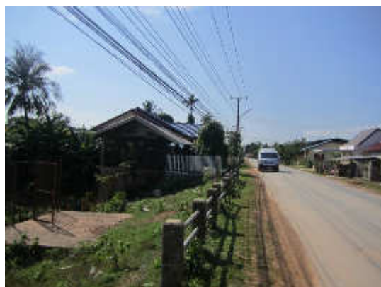
View of the road where Houay Nam Sot and the floodgate are located.
