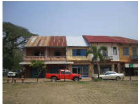
Figure 20: Current condition of Old Post Office Building
