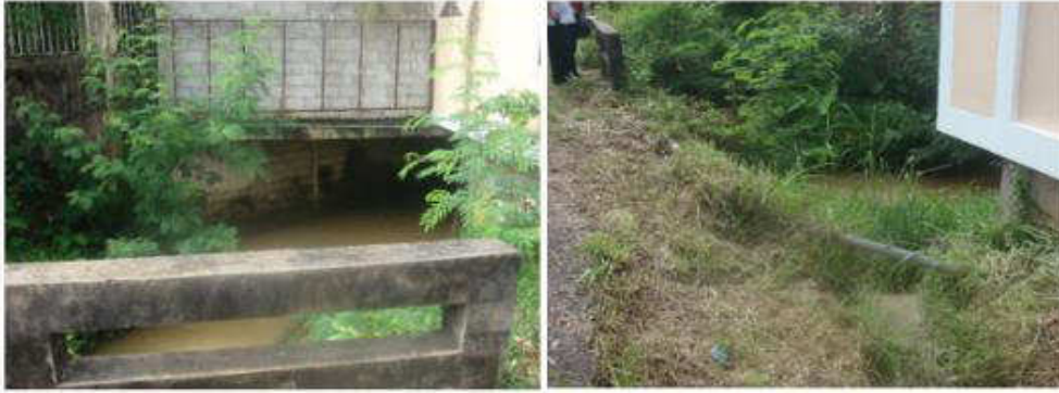
Drain C Structure over and utility lines adjacent to the drainage courses
