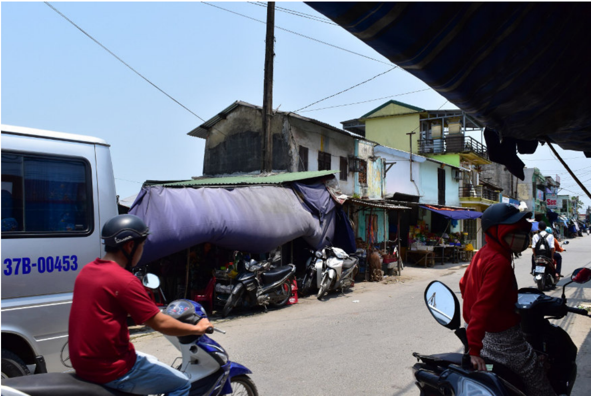
The affected House-Cum-Shop at Bao Vinh Pier
