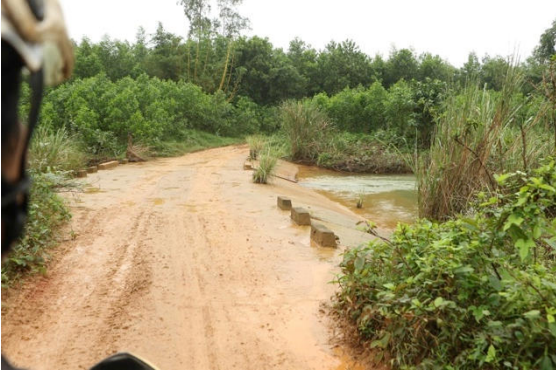
Stream crossing at Km11+882.07
