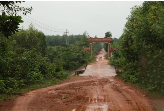
View to Trang Rong gate & the existing spillway
