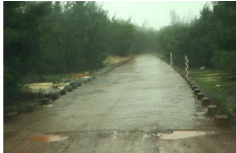
Spillway at Km3+512 - Section 1
