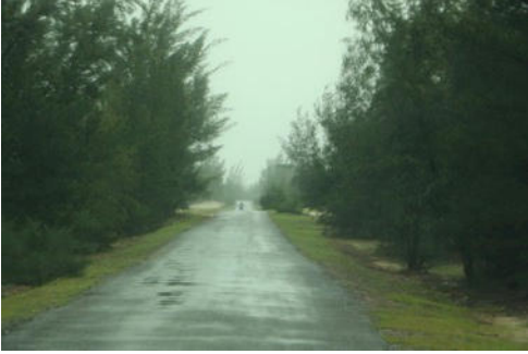
A good road section in Section 3
