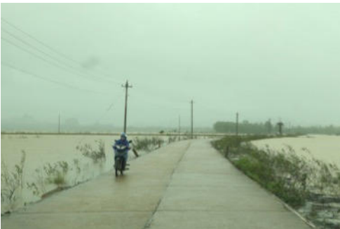
Flooded rice fields along Section 2 of the road
