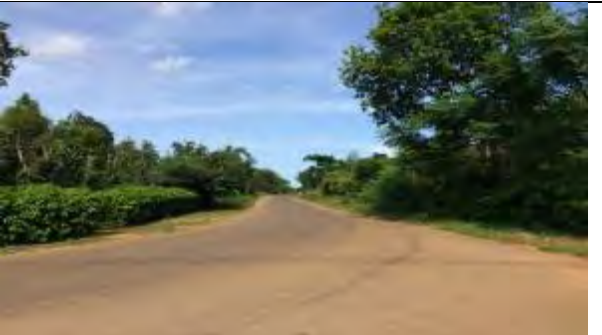
Section 1: end point at Km8+061
