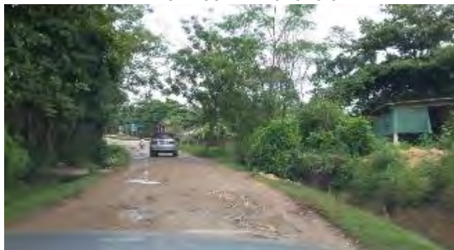
Km10+00: road surface degraded with large potholes
