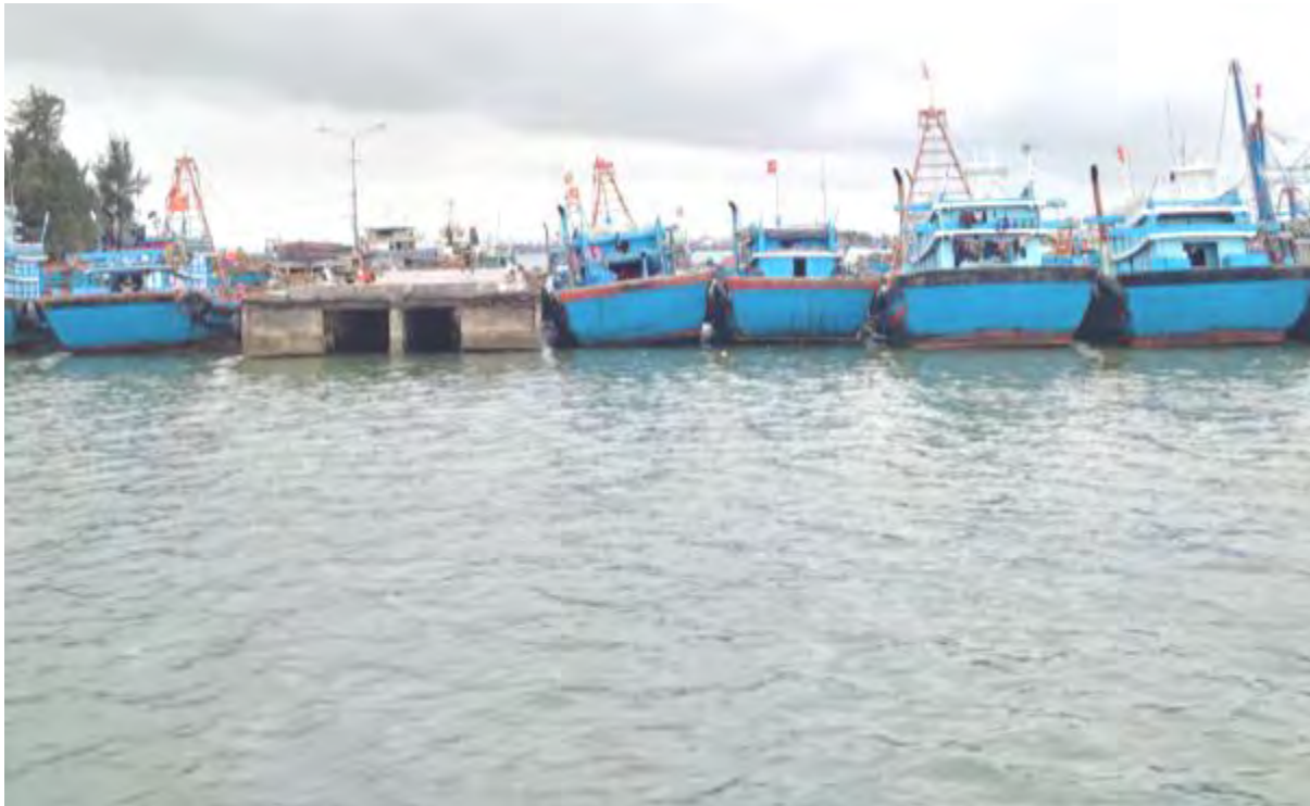
Figure 3: Existing status of the waterfront in front of the wharf is deposited and there is no signal buoy
