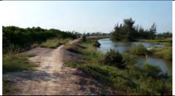
Earth embankment alignment along the canal and mangroves
