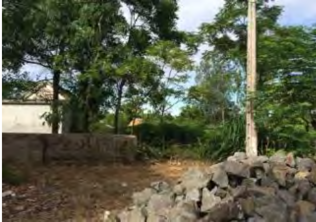
Km0+170: location to cut new (alignment) road
