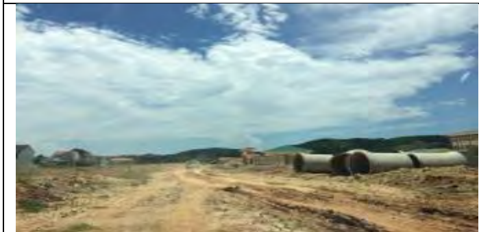
Section 1 – Road N7, Km0+900
