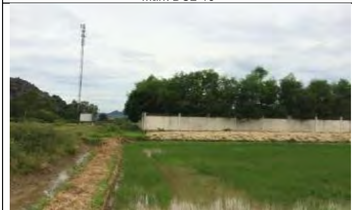
The road alignment goes through the fence of the school at Km7+400
