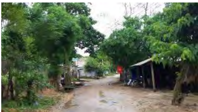
Km4+00: degraded with water drainages and potholes through the residential area
