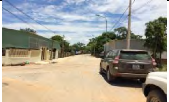
Section 1 – Road N7, Km1+200
