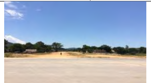
Section 1 – Road N7, Km0+600
