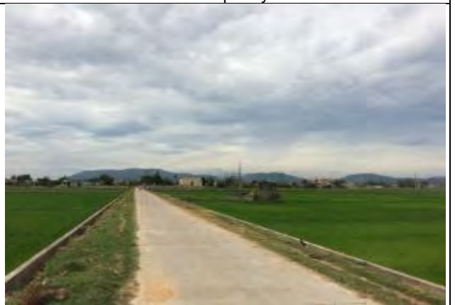
Intersection point with cement concrete road at Km0+300
