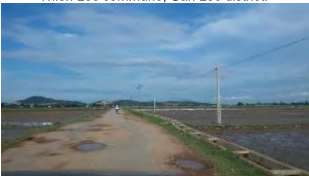
Km 1+685: earth road with large potholes and irrigation canal along the road
