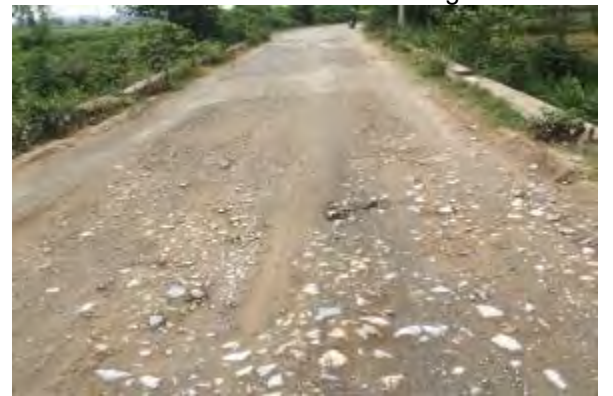
Km4+750: road section above culvert
