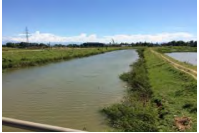
Km1+350 Gach Ngoi bridge
