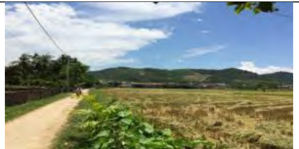
Section 1 – Road N7, Km0+400
