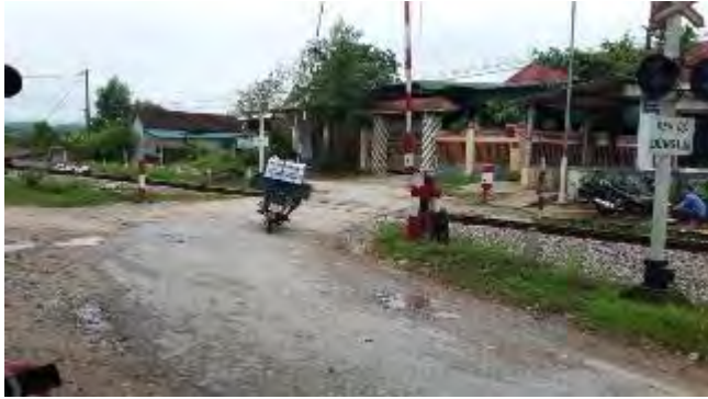
Km7+877: intersection site with the railway
