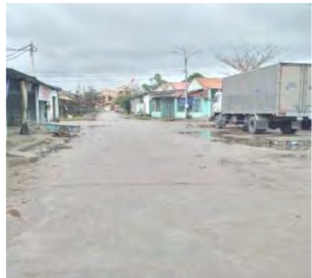
Figure 6: Existing status of the road system: waterlogged, degraded
