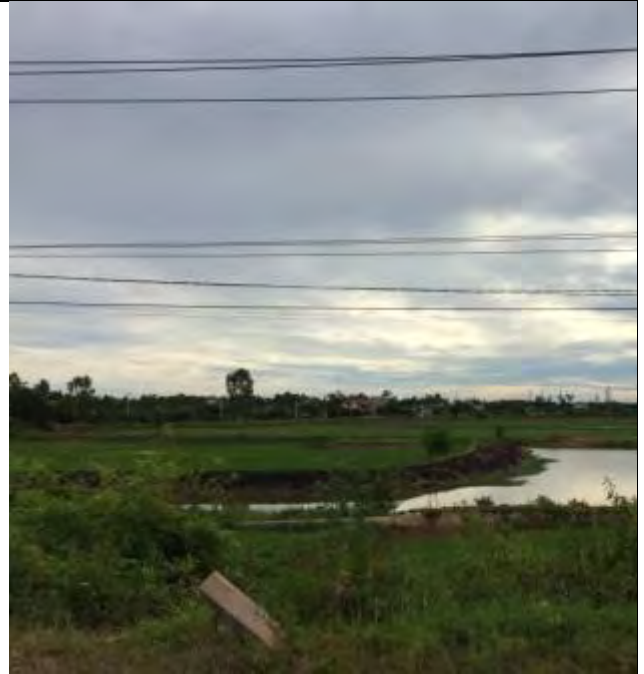
Xom Zet bridge construction site at Km4+200
