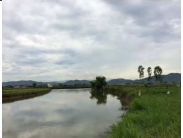
Thuan Loc bridge construction site at Km2+700
