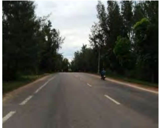
Starting point at Km0+0.00 connecting to Truong Phap street
