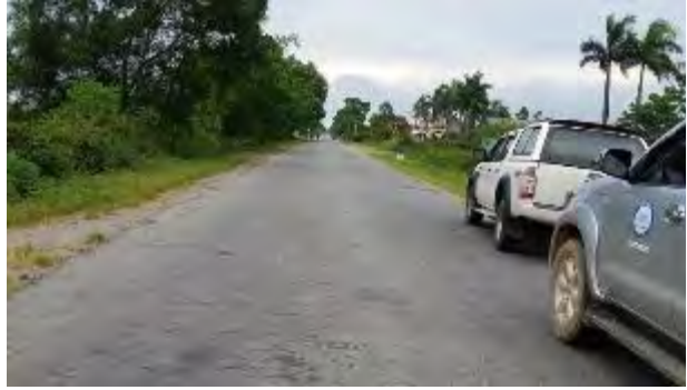
Intersection point of PR546-Km1+500
