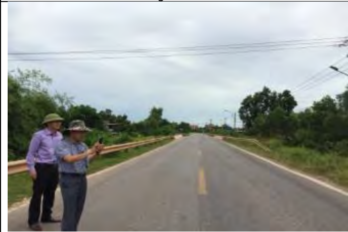
End point at Km4+298,84 connecting to HCM road
