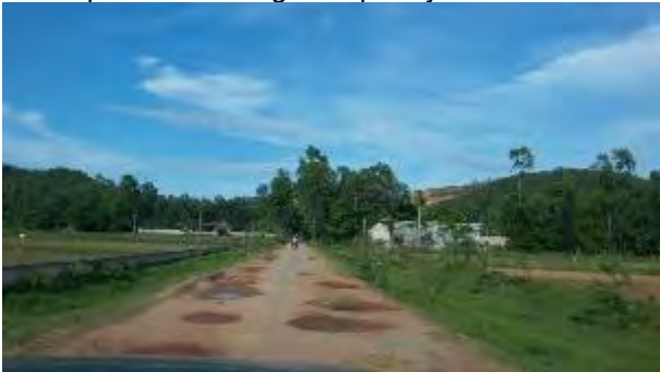
Km 5+00: gravel and earth road with large potholes
