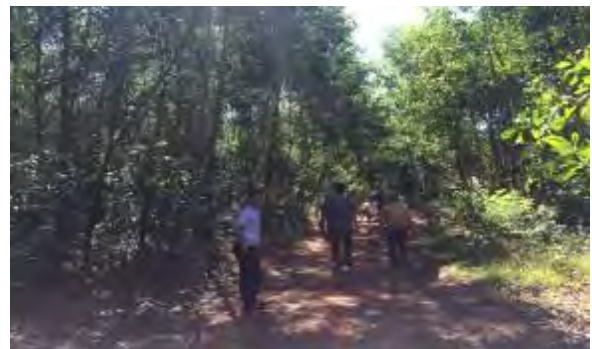
Existing road at Km0+350
