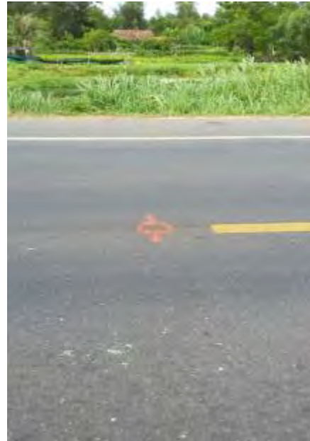
Mark point at Km0+0.00: central line of NH1A
