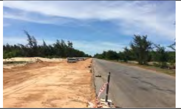
The existing ongoing construction works subproject connected to the proposed road subproject Road#1:
