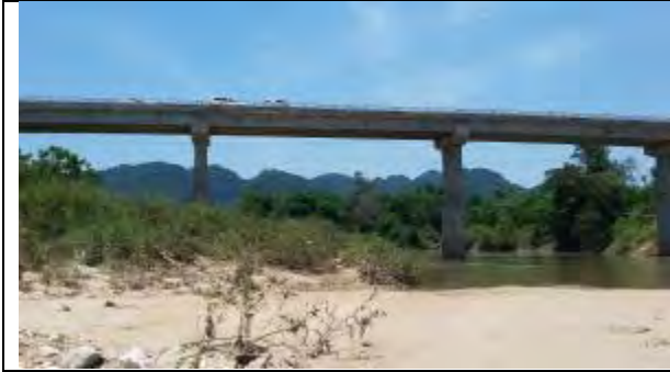
End point of Quay Chau Embankment connects to Quay Chau bridge
