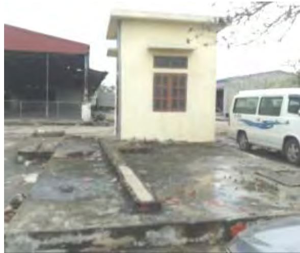
Sewage treatment plant 30 m 3 / day-night
