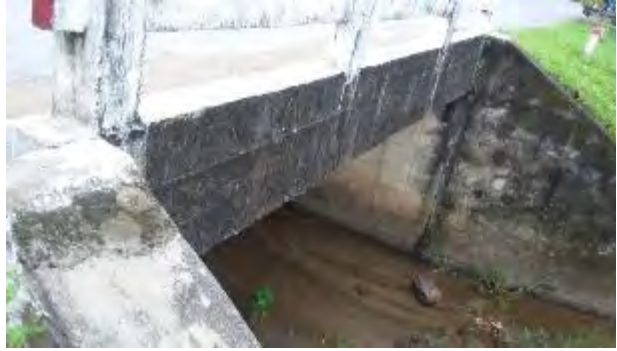
Km6+903: My Thanh bridge seen from below
