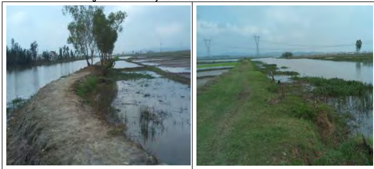
Figure 3: Culverts and Gated Culverts
