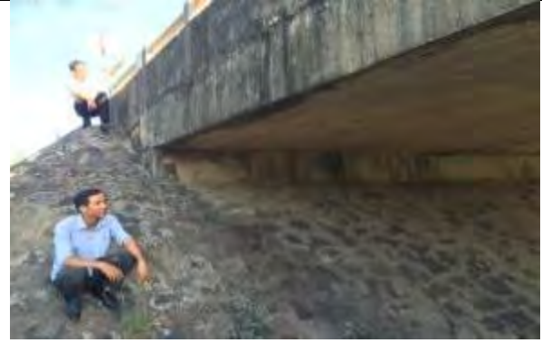
My Chung bridge Pier on PR576b
