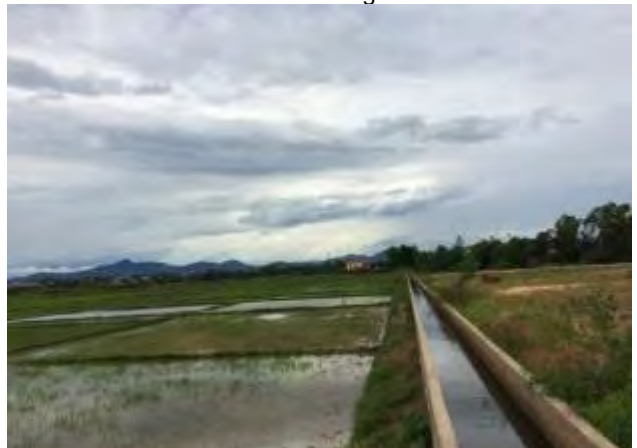
Km2+900: rice irrigation canal
