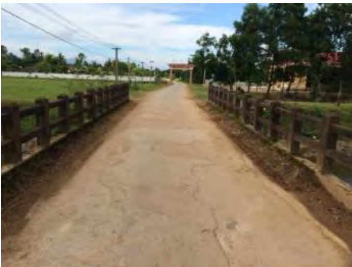
Km1+550+0.00: Liên Tân bridge surface site
