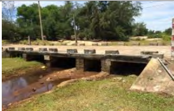
Section 3 at Km4+260 (existing culverts)
