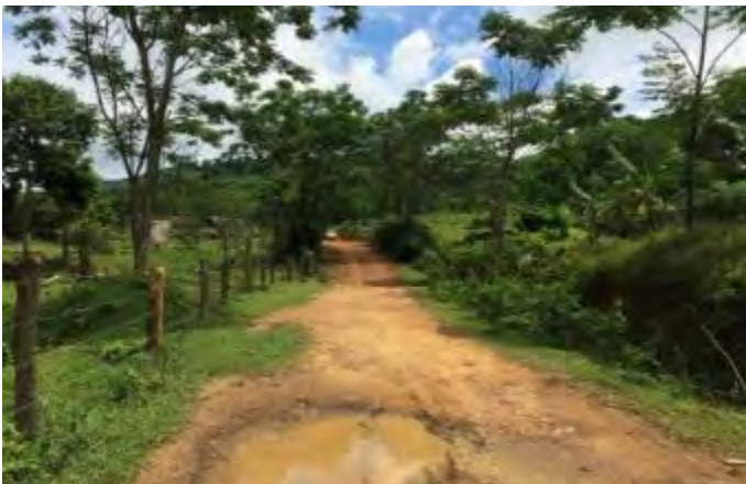
Km13+700: existing earth road surface with large pothole
