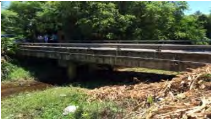
Co Luy bridge Km8+003
