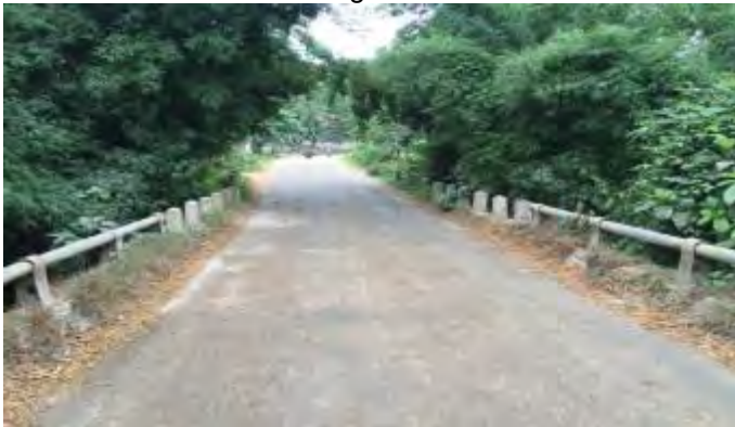
Km1+765.50: Am bridge
