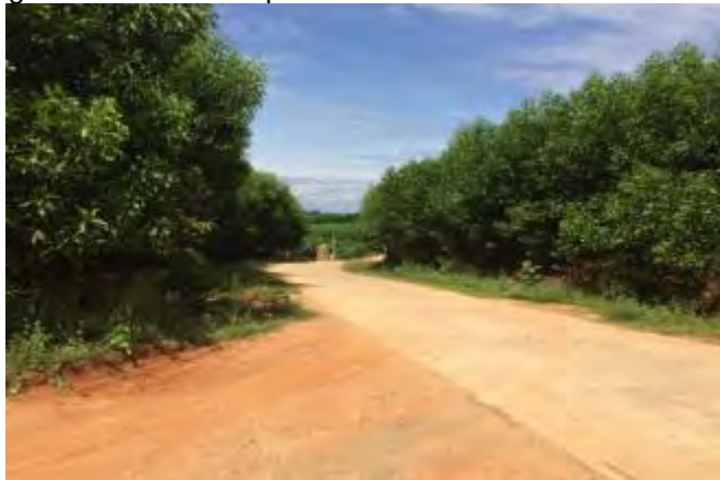
Km3+750.00: location intersecting with the cement concrete road
