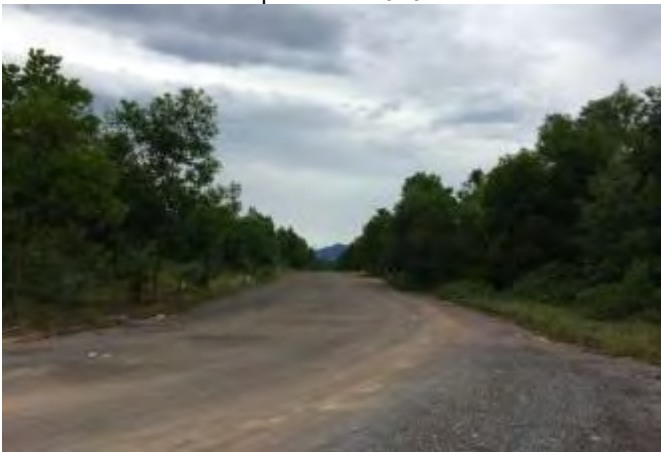
End point at Km3+817: the road connects to the ring road of Tay Bac industrial zone in Dong Hoi city
