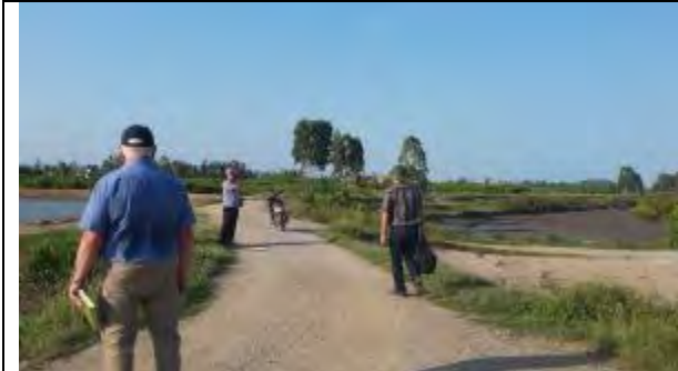
Earth surface embankment
