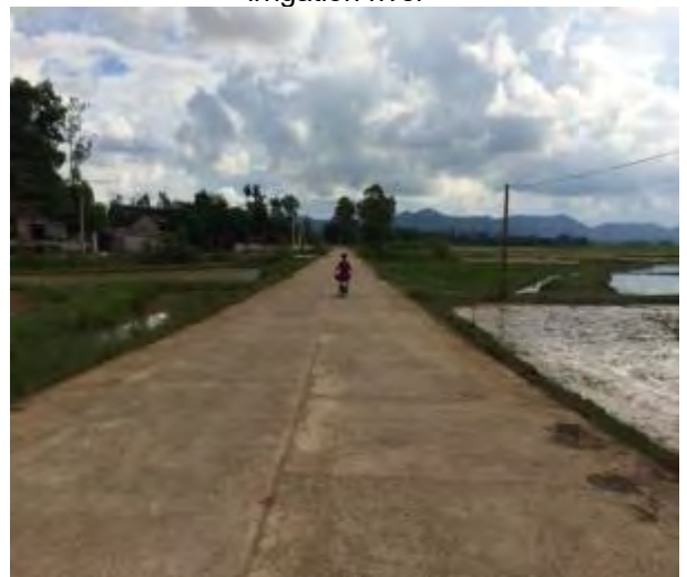
Km1+575: intersection site with the existing spillway
