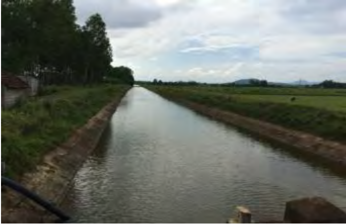
Km1+550+0.00: Lien Tan bridge surface
