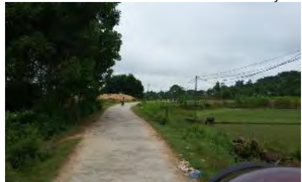
Km8+500: asphalt concrete road narrow width of 3,5m
