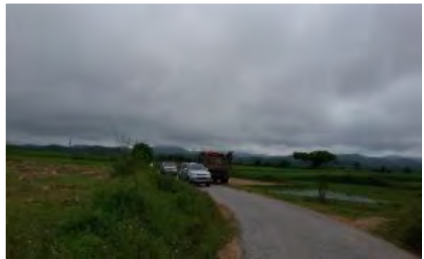
Km6+500: asphalt concrete road narrow width of 3,5m
