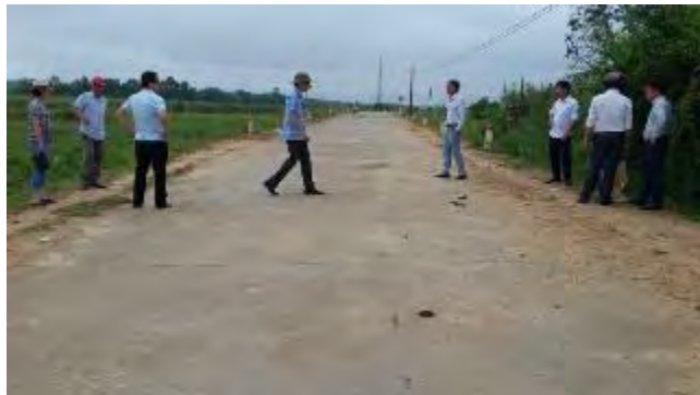
Km2+074: end point of section 1
