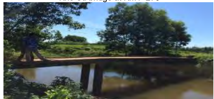
Existing bridge at Km1+270
