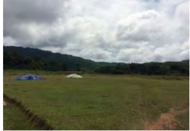
Km14+00 new alignment / road goes along the stream uphill
