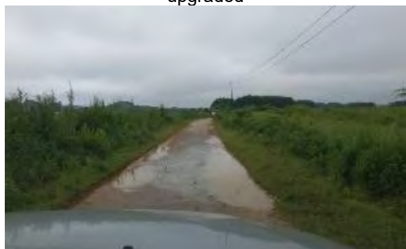
Km3+00: degraded gravel road section with large water pools and potholes on both sides
