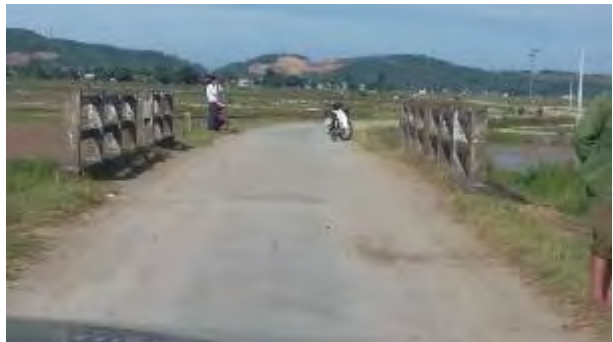
Km 0+ 750: bridge#1 in poor and damaged condition
