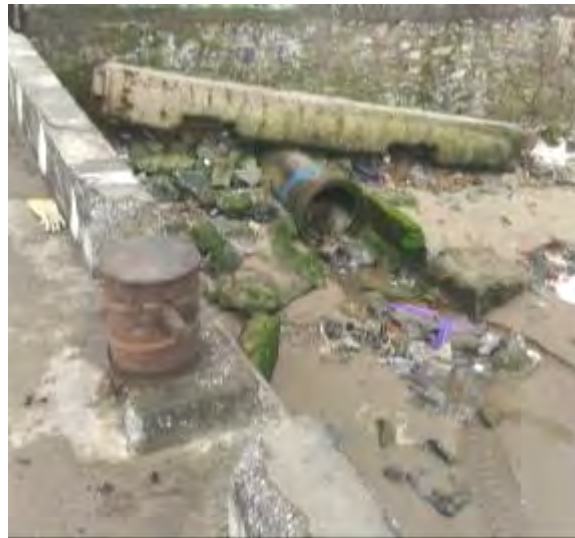
blocked sewer drain
