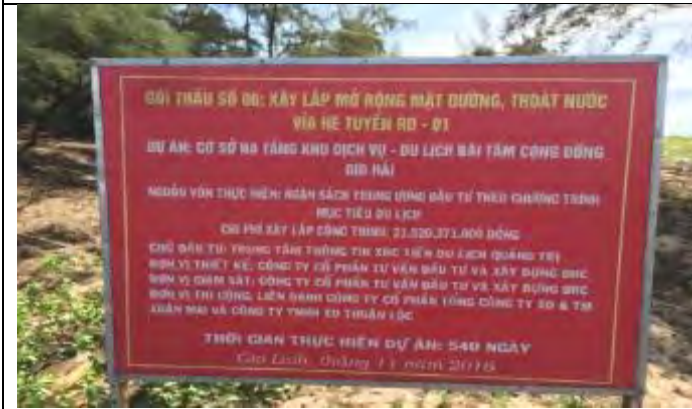
Gia Hai Tourism Service project ongoing construction works
