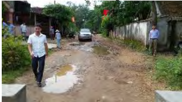
Km2+480: connection point of the road to bridge
