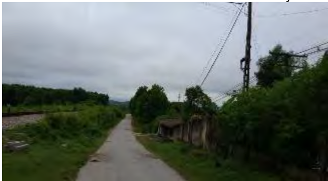
Km7+900: asphalt concrete road narrow width of 3,5m
