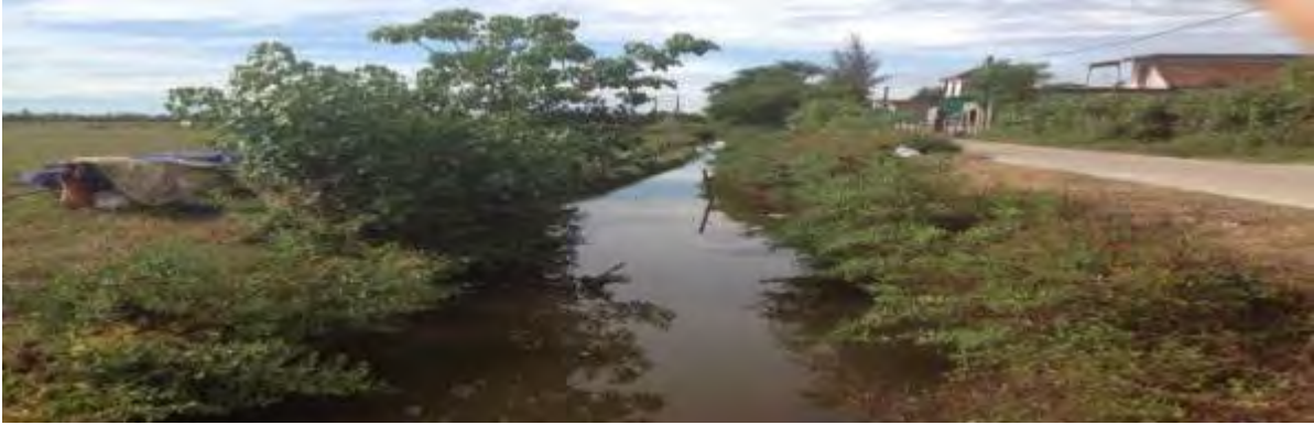
Status of drainage channel in Ho Do commune
