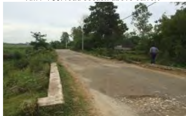
Km6+800: damaged road surface
