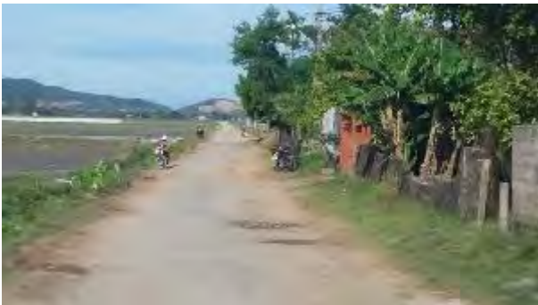
Starting point at Km0+00: Adjacent to asphalt road (on district road 3) in Tan Thuong hamlet, Thien Loc commune, Can Loc district.
