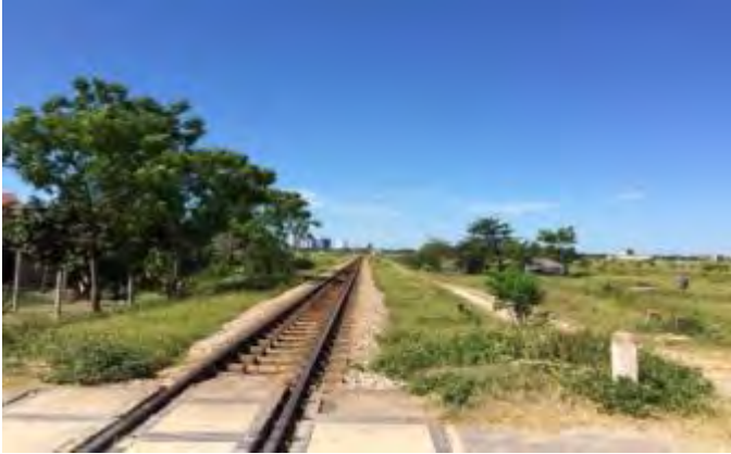
Railway crossing point at Km3+00
