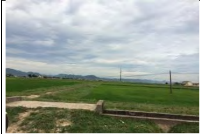
Km0+120: rice irrigation canal
