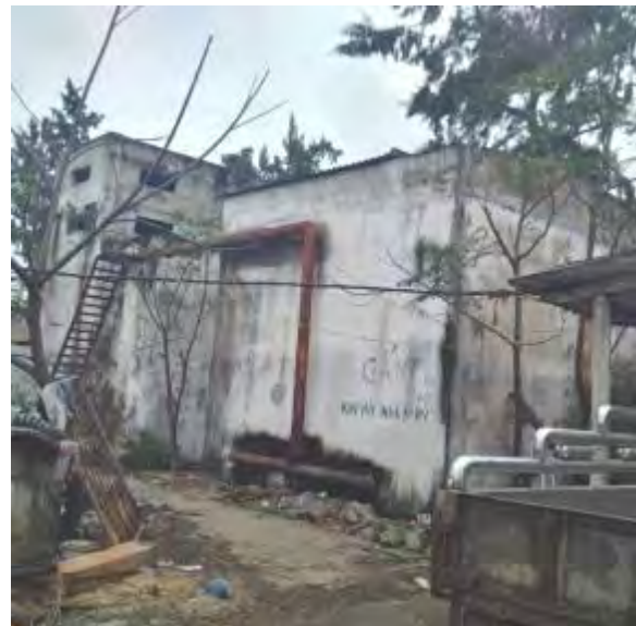
Broken sediment filter
