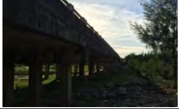
My Chung bridge on PR576b
