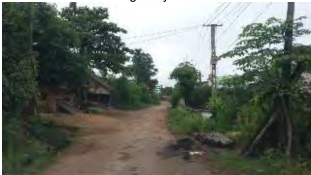
Km1+600: degraded gravel road through the residential and garden group areas
