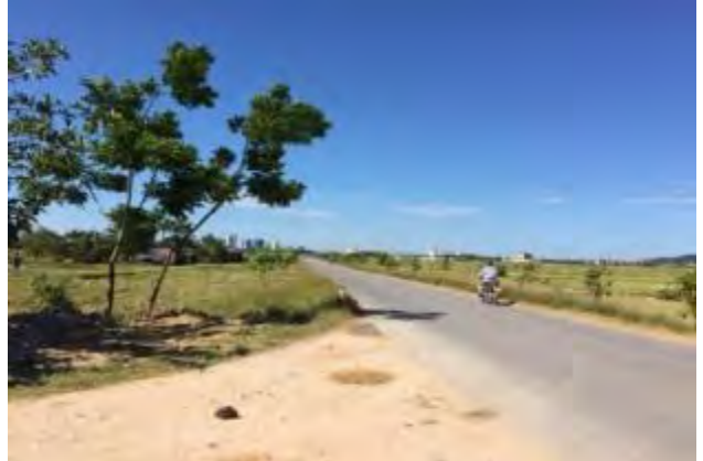
End point connecting to NH8B - Km3+80 .00
