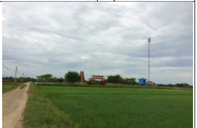
The road alignment goes closely along the cemetery Quang Tan at Km3+100
