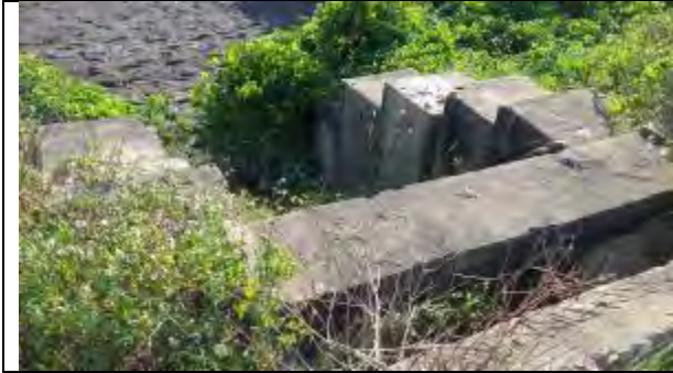
Damaged Drain culvert
