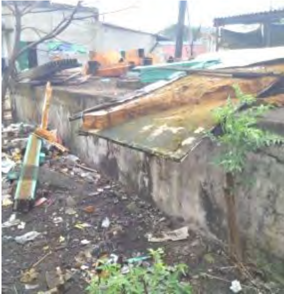
Degraded water tank of 160 m 3
