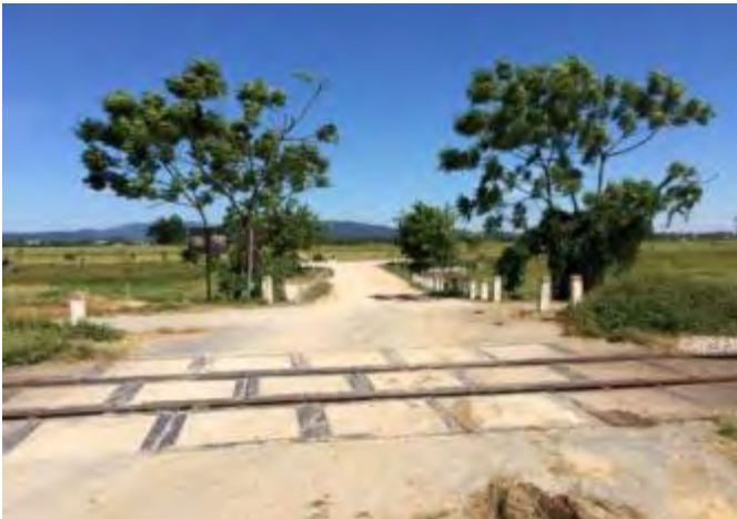
Railway crossing point at Km3+00
