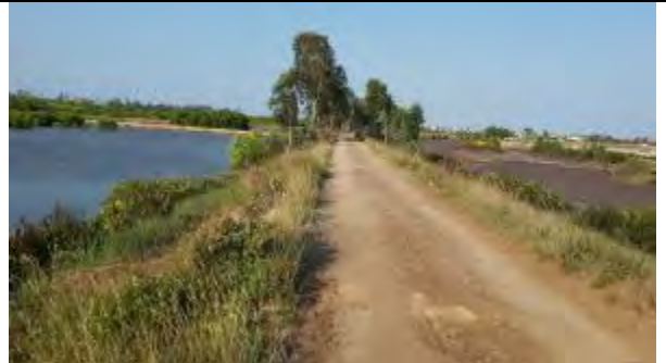
Earth surface embankment
