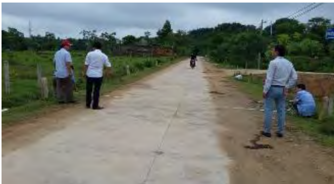
K9+926.9: starting point of section 3 upgrading the road before the world bank funded road project from km7+877.38 to km9+926.9
