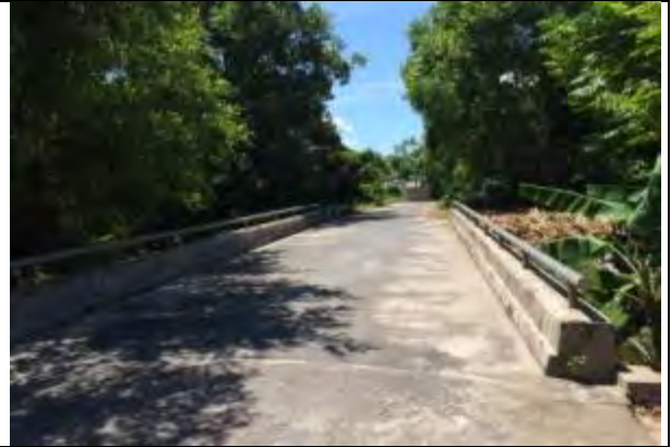
Co Luy bridge Km8+003
