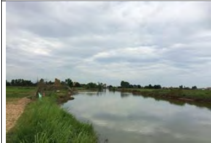
Thuan Loc bridge construction site at Km2+700
