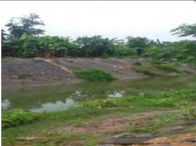
Km:2+300: new bridge to be constructed over the river
