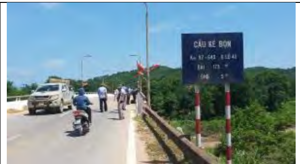
Starting point of Quy Chau Embankment at Ke Bon bridge
