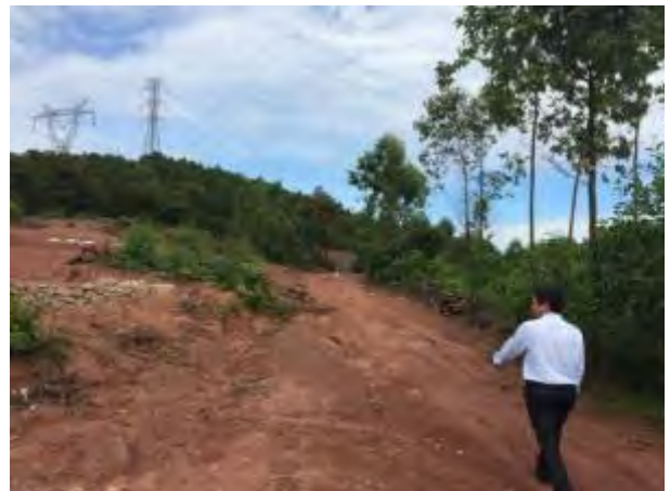
Km0+800: new road location
