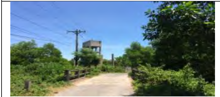
Box culvert Km12+170
