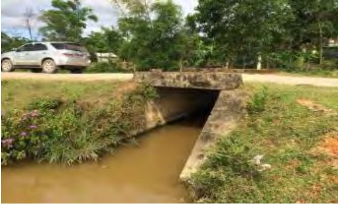
Slab culvert site at Km2+500
