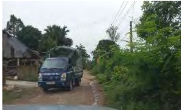
Km1+450: degraded gravel road through the residential and garden group areas
