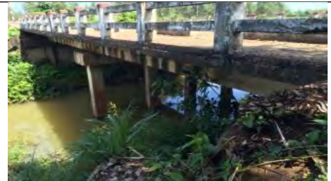
Section 1 at Km3+160 (Duc bridge)
