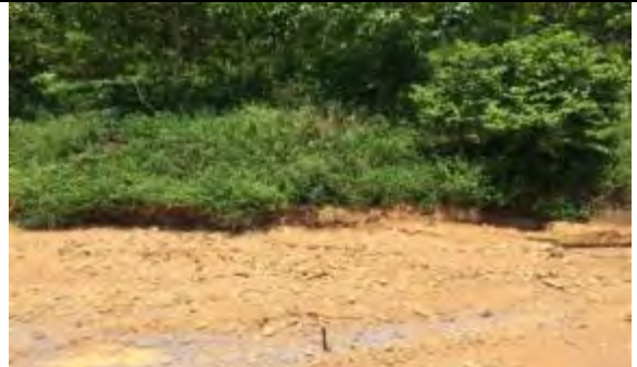
Section 2 End point – Km0+620 connecting to N8
