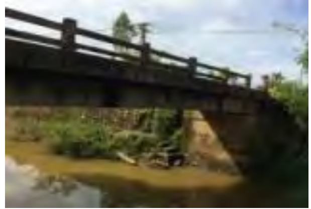
Km0+555: Rọc Cắn bridge site taken from below
