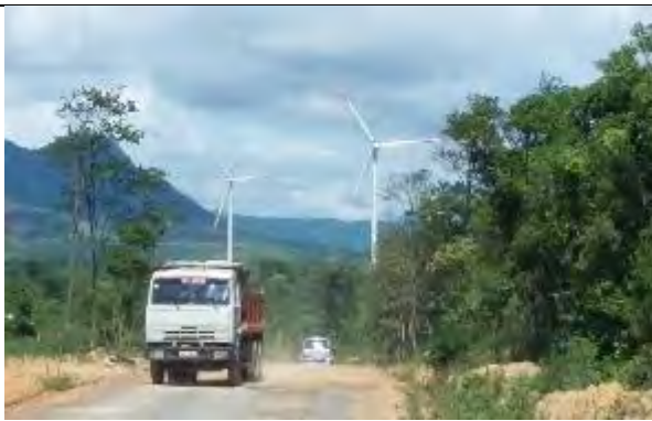
Wind power Turbines
