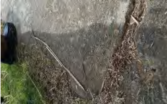
Km4+200 starting point of new alignment
