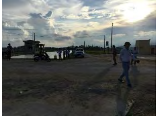
Ending point at km10+00 connecting to provincial road 547 (at Petro station in An Loc commune, Loc Ha dist.)
