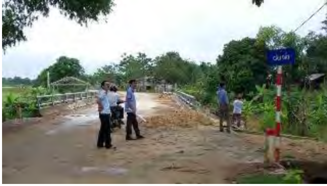
Km5 + 053.24: Dat bridge with a span of 8m, 15m long was constructed in 2016
