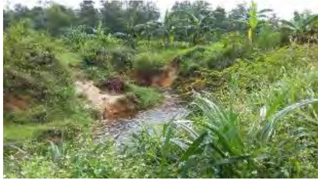
Km0+800: stream and ecosystem on the left side of spillway crossing over the road
