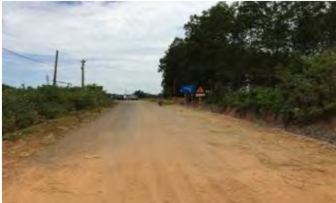
Section 1: End point at Km2+150
