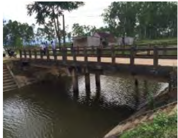
Km1+550+0.00: Liên Tân bridge left side
