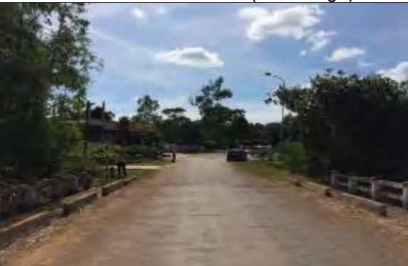
Section 1 at Km3+200 (Duc bridge)
