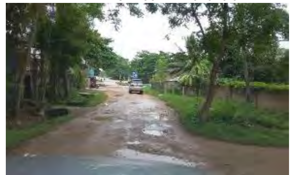
Km10+300: road surface degraded with large potholes
