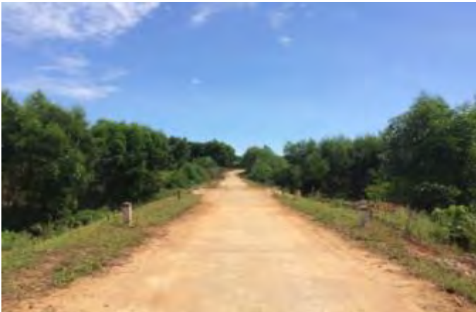
Km4+150.00: existing culvert location on the cement concrete road
