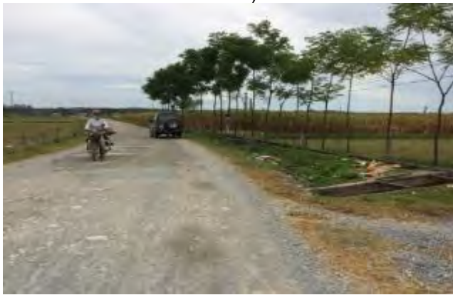
Km1+0.00: irrigation culvert site
