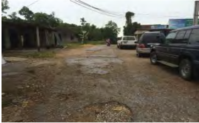
Km10+100: degraded road surface
