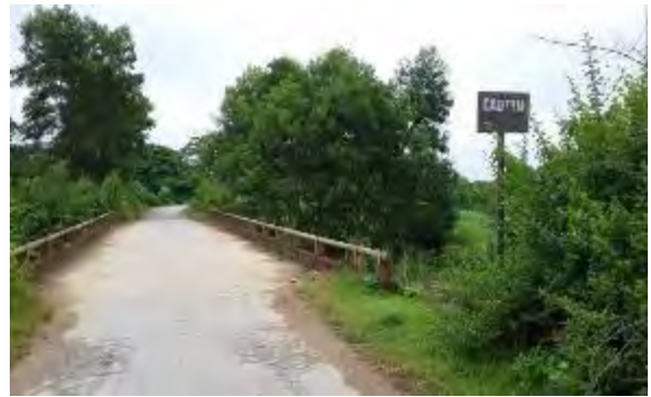
Km5+800: Tan bridge (constructed in 2003) is deteriorated
