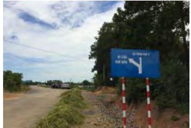
Section 1: End point at Km2+150
