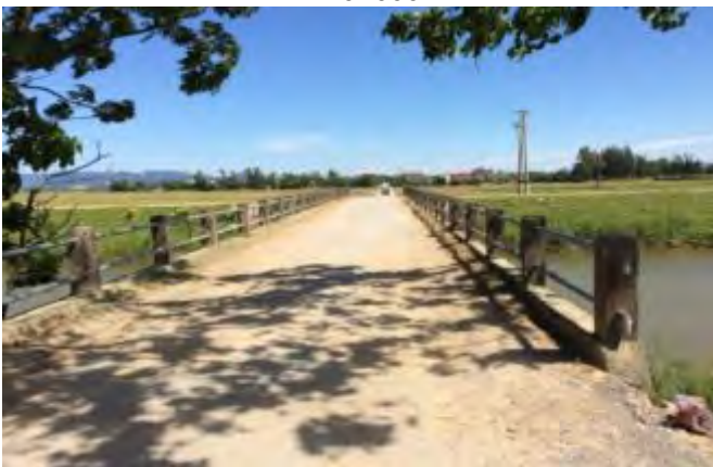
Km1+350 Gach Ngoi bridge
