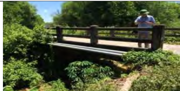
Box culvert Km12+170
