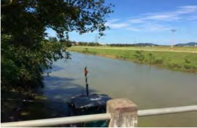
Km1+350 Gach Ngoi bridge
