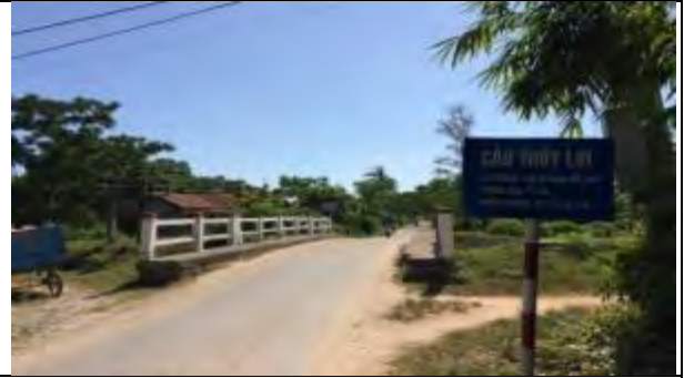
Existing bridge Km1+458
