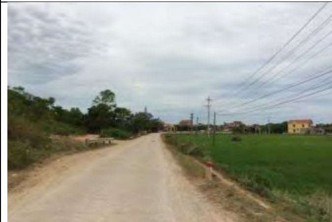
End point Km9+775, intersecting with PR559
