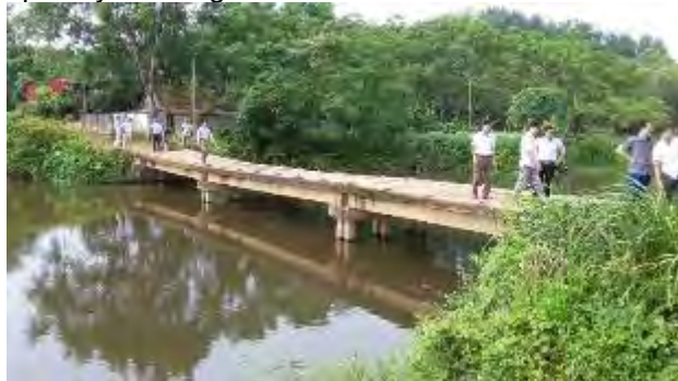
Km2+480: poor bridge status
