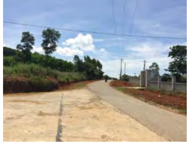
Km5+100: Intersection point with DR143
