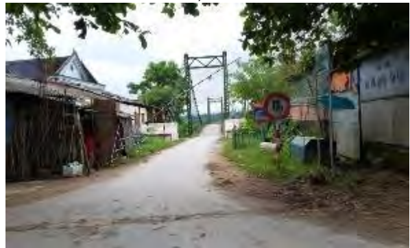
Km7+877: fly bridge load design 10T
