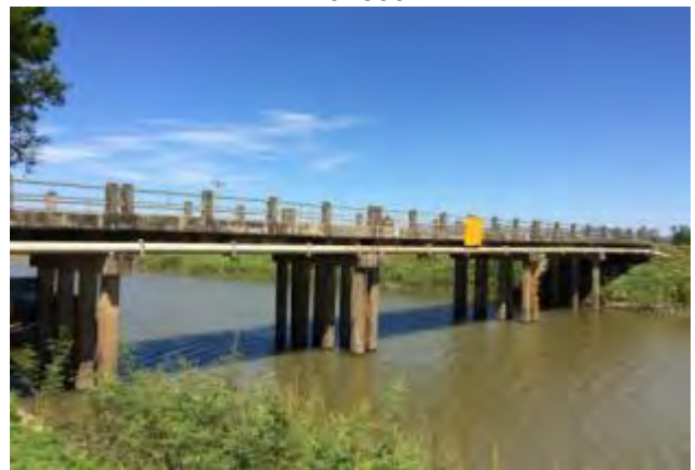
Km1+350 Gach Ngoi bridge
