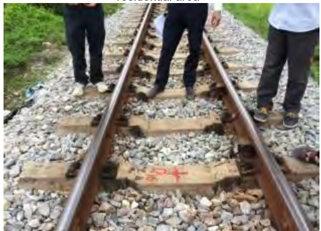
Railway crossing point at Km3+125
