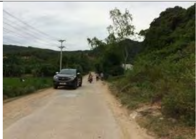
End point Km9+775, intersecting with PR559
