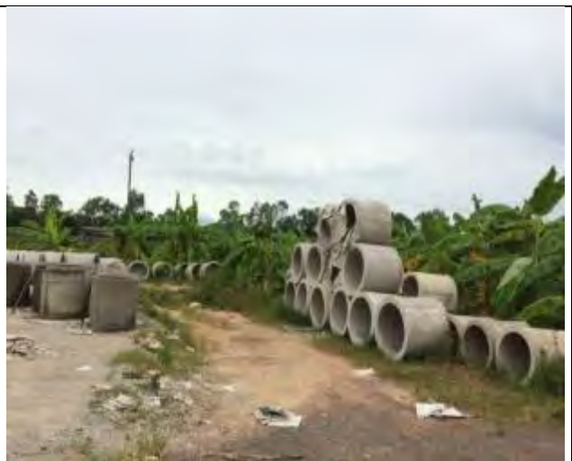
Km0+30.00: the new alignment goes through the garden and rice fields
