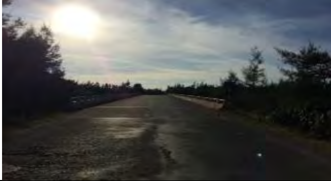
My Chung bridge on PR576b
