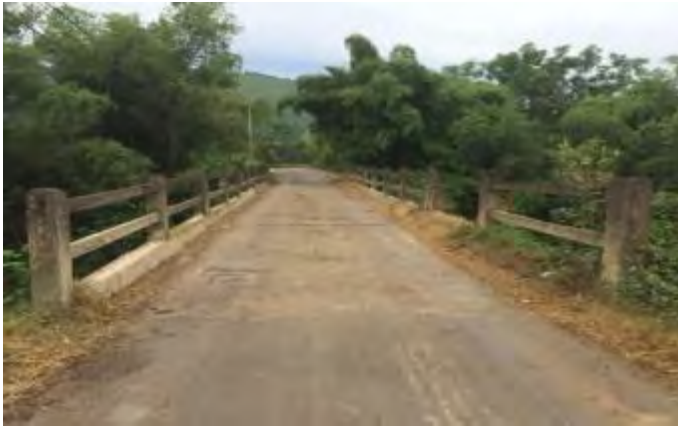
Km4+179.66: Hoi Met bridge deck and surface
