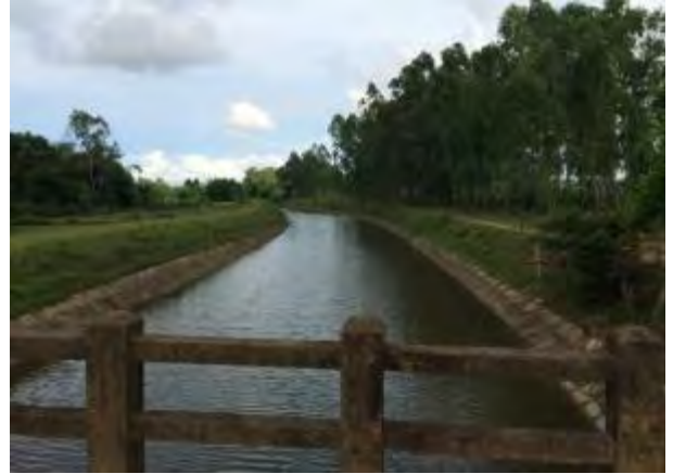
Km1+550+0.00: Lien Tan bridge over the irrigation river
