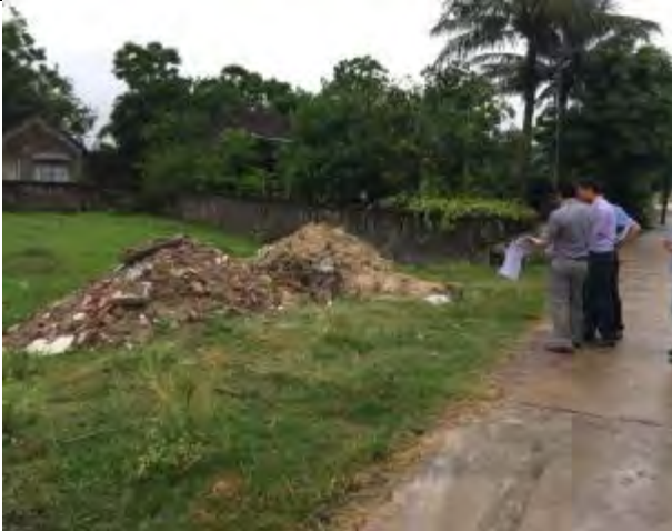
Km:2+100: new alignment road through the residential area
