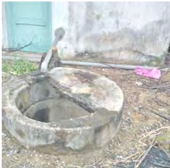
Unusable groundwater well
