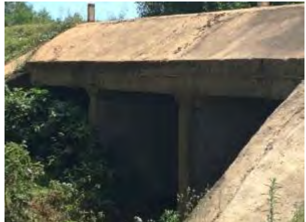
Km4+150.00: existing culvert location on the cement concrete road
