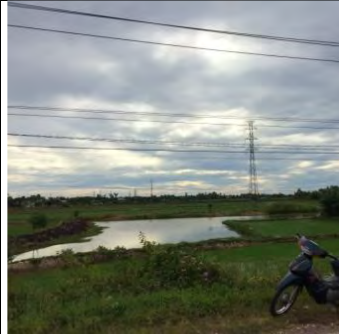
Xom Zet bridge site at Km4+200
