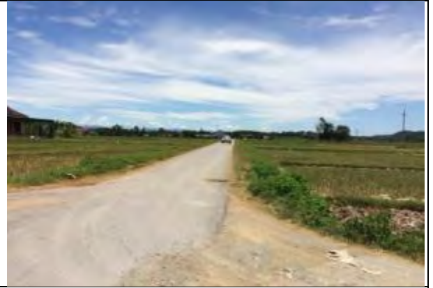
End point: Km8+200
