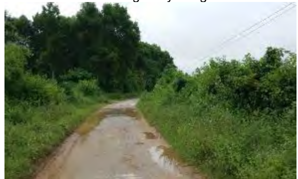
Km3+300: degraded road surface with large water drainages both sides and acacia trees on the left side of the road
