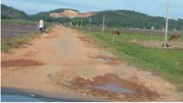
Km 2:500: gravel and earth road with large potholes through the paddy field area
