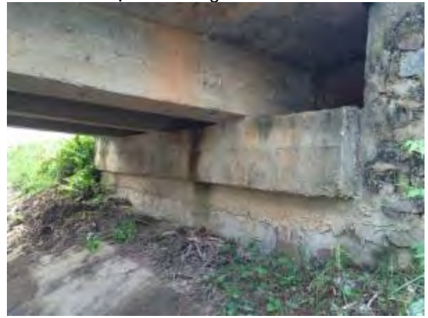
Km0+555: Rọc Cắn bridge site taken from underneath
