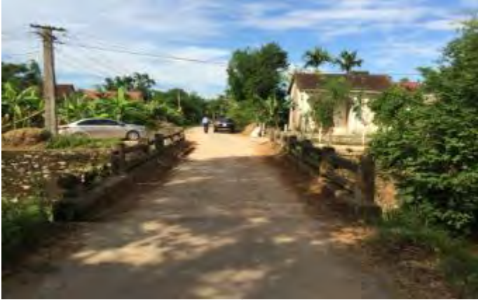
Km0+555: Rọc Cắn bridge location
