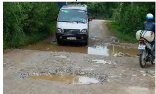
K9+926.9: starting point of section 4 upgrading the road after the world bank funded road project from km7+877.38 to km9+926.9
