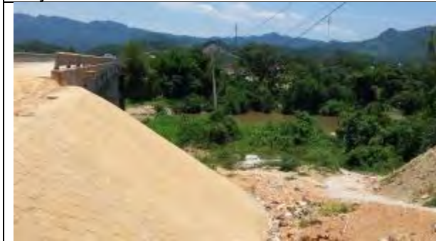
End point of Quy Chau embankment connects to Quy Chau bridge
