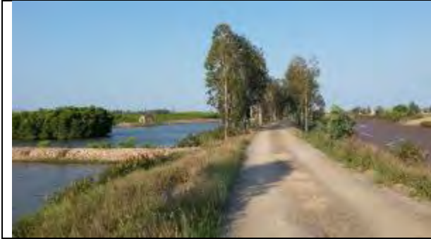
Earth surface embankment
