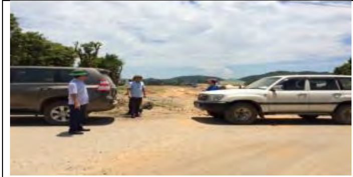
Section 1 – Road N7, Km1+200
