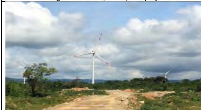
Wind power plant at Km11+500
