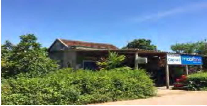
End point at Km2+160 connected to PR579
