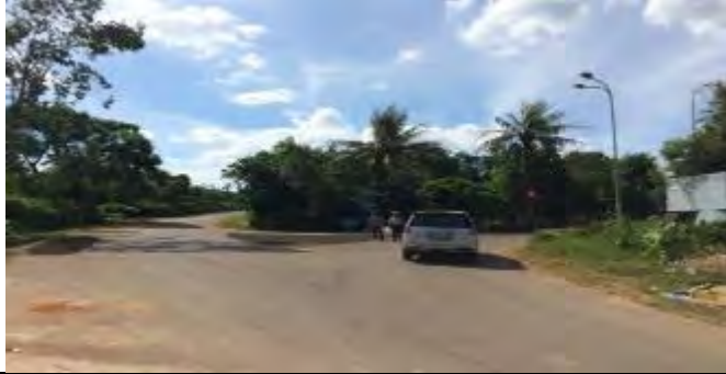
Section 1: T-junction of Duc bridge at Km3+240
