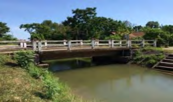
Existing bridge Km1+458
