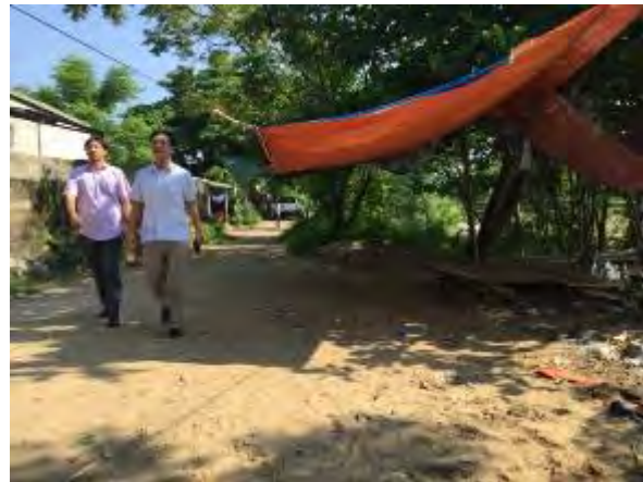
Village 17 of Phúc Thọ commune (The dyke is located outward and adjacent to the riverbank)
