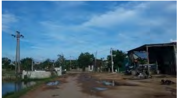
Km6+450: road surface seriously degraded with big potholes
