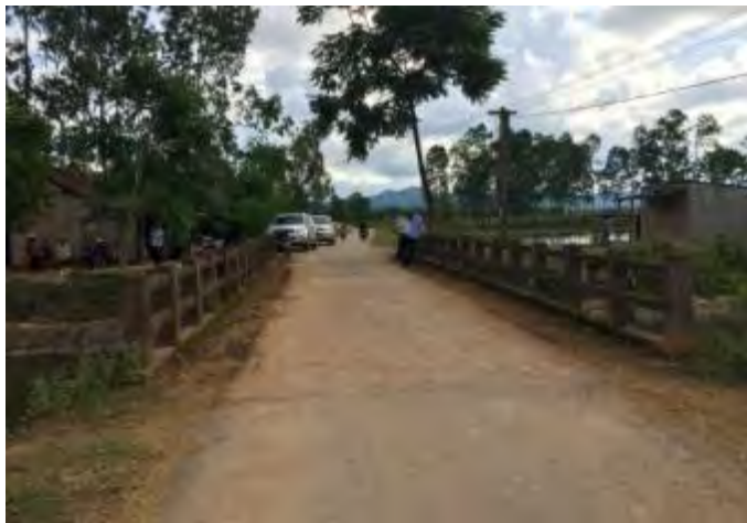
Km1+550+0.00: Liên Tân bridge surface site
