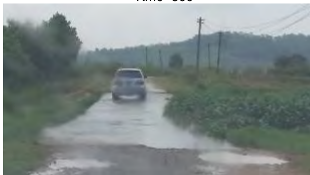
Km0+800: spillway crossing over the road
