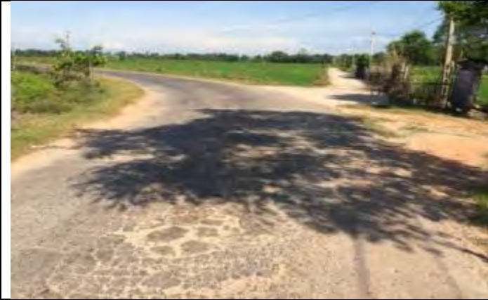
Existing road surface cracked Km1+500
