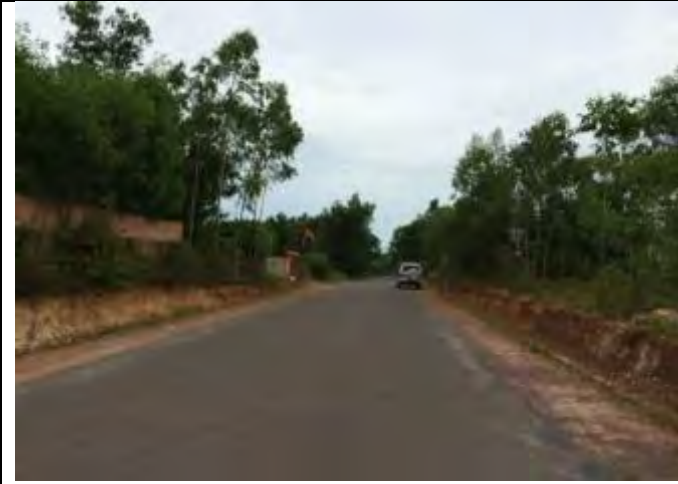
Intersection point with the asphalt road at Km2+850
