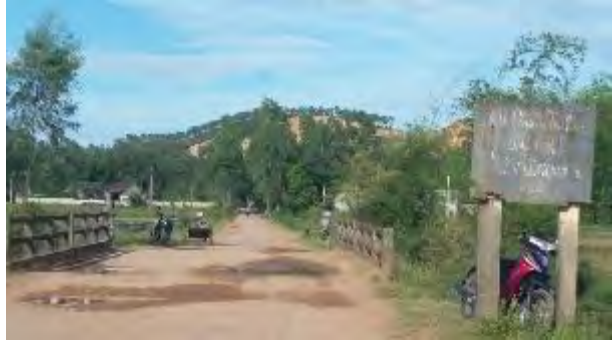
Km 3+720: bridge#2 seriously degraded condition
