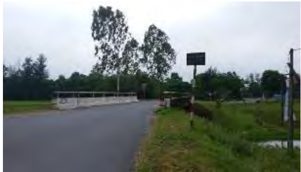
Xuan My bridge at Km6+229
