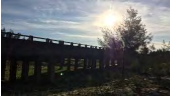
My Chung bridge structure on PR576b
