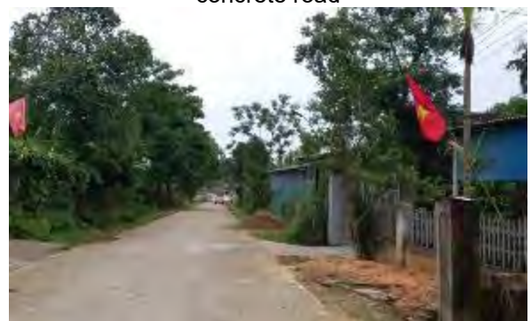
Km4+852: End point of section 2
