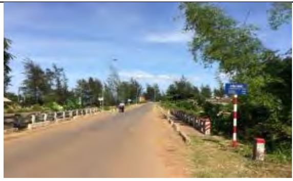
Section 1 at Km3+160 (Duc bridge)
