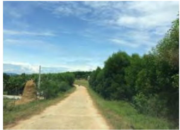
Km4+100: cement concrete road
