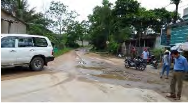
End point at Km10+361,12 connects to HCM Trail at Km824+800 road surface degraded with large potholes
