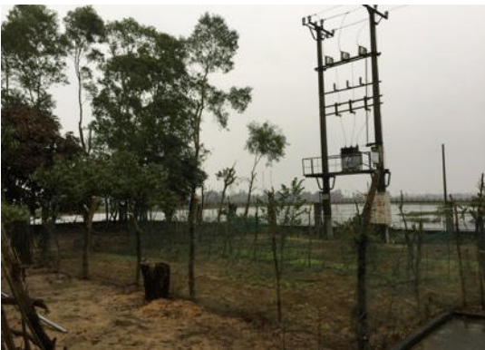
Location for water tank in booster station
