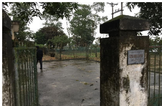
Proposed site for the booster unit to connect to the two Ha Tinh city WS plant
