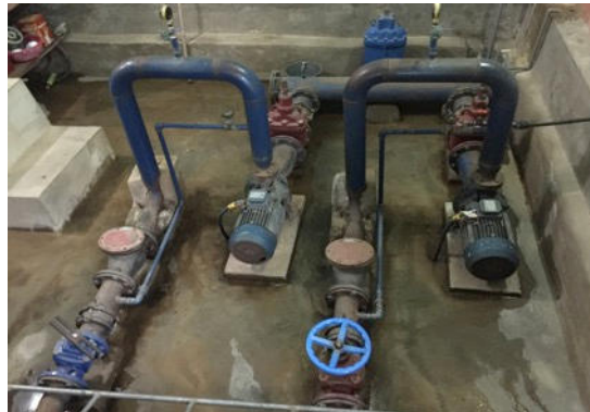
Current pumping system of Thach Ha booster station
