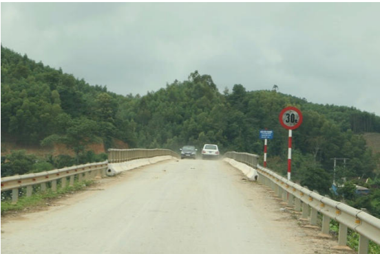
The Existing Cay Chanh Bridge
