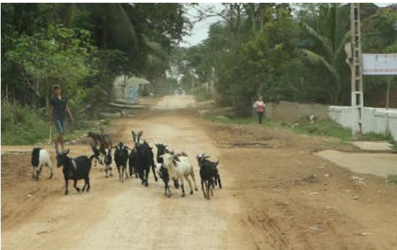
Damaged asphalt road section
