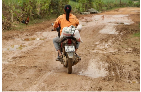
A bad road section
