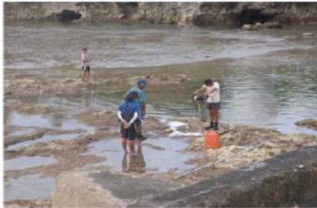
Plate 1 study site, Niue, Alofi fringing reef – drilling adjacent to Sir Roberts Wharf at low tide. Topographic survey 10th - 24 th May 2013.
