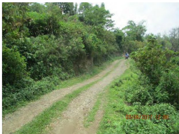
Photograph 1. Start point (15+000 chainage). Note the Sasidhar Nirwan sewa has finished the earthworks and back cutting of the proposed road from 10+000-15+000. From this point the works need to be done.
