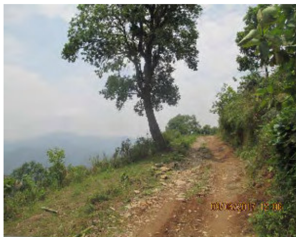
Photograph 2. The typical alignment of the road at ch 15+450. Note the road needs widening and proper drainage system.
