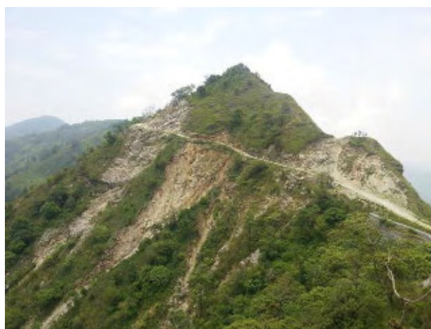
Photograph 4. Start of the steepest (20+400-20+700) of the road. Note the area is critical for landslide and need proper slope stabilization.
