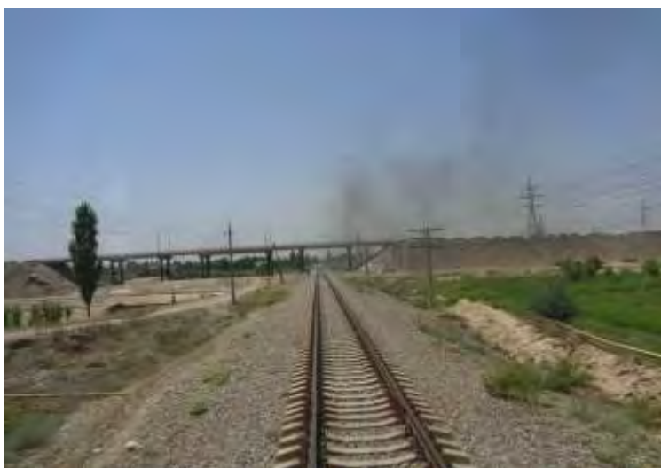
Figure 31: Existing situation - emission of carbon deposit from diesel locomotive
