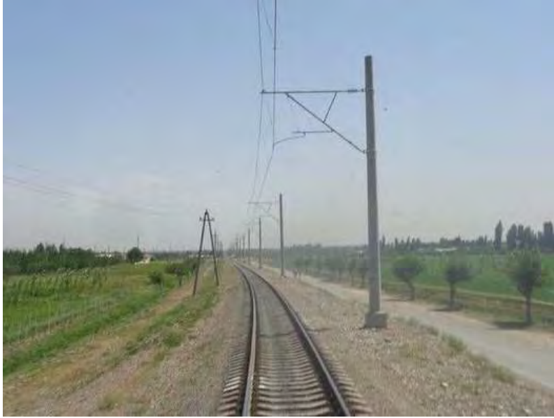
Figure 4: View of contact-system masts (picture from operating Andijan-Kokand railway)
