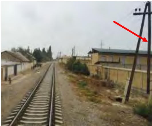
Figure 5: Existing 10 kV OHL
