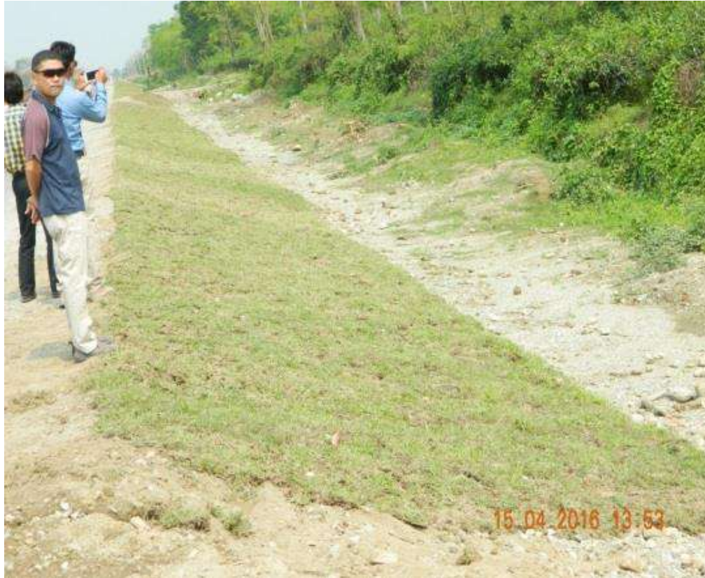
Photograph 8: Turfing work on the slope of the Embankment (AH-48)
