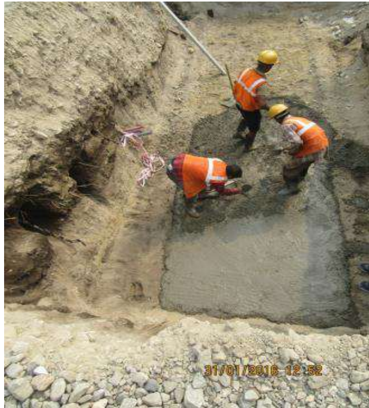
Photograph 10: PPEs and Safety Measures are Provided to the workers (AH-02)
