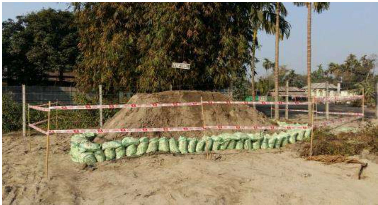
Photograph 5: Topsoil is preserved for reuse at campsite of Rangali Bazna (AH-48)
