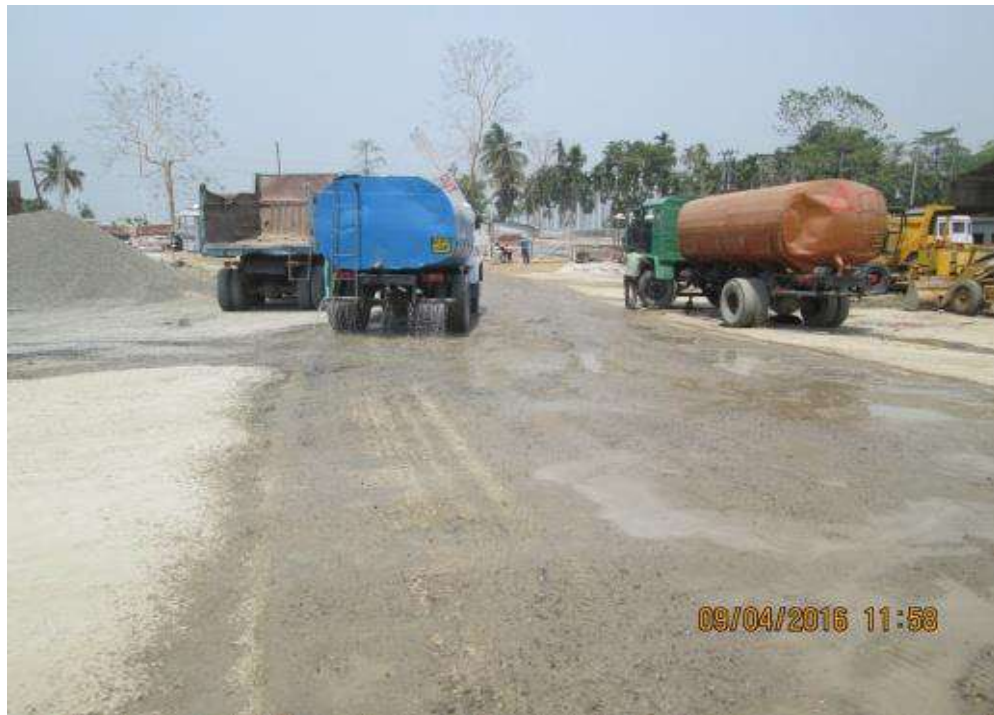
Photograph 6: Sprinkling of Water on AH-02 Subproject
