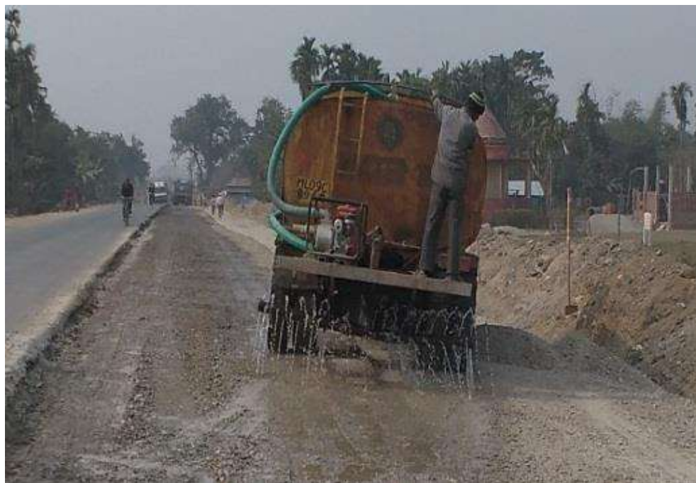
Photograph 7: Sprinkling of Water on AH-48 Subproject
