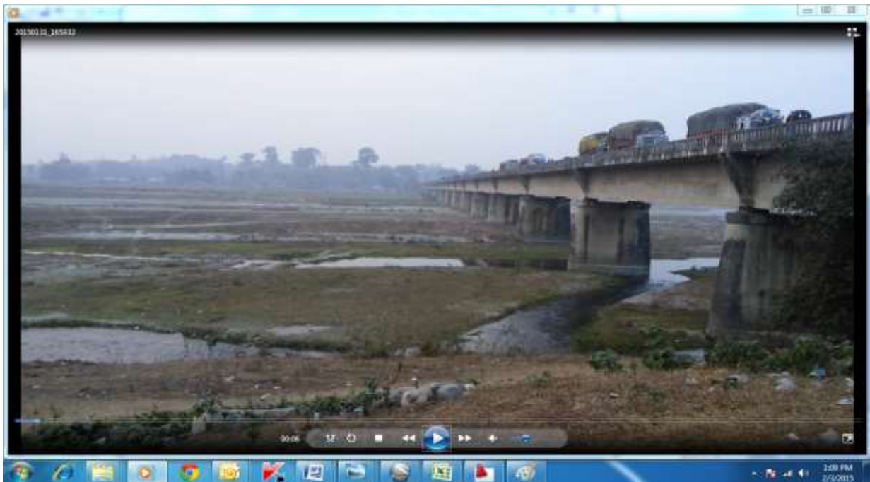
Figure 14: View of river at the existing bridge
