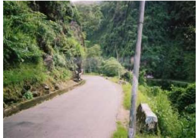
Image 8: Landslide Prone Location along Imphal-Moreh road
