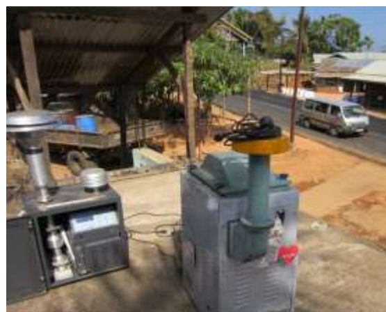
Image 5: Air Quality Monitoring Station Setup at Wanjing (AQ2)
