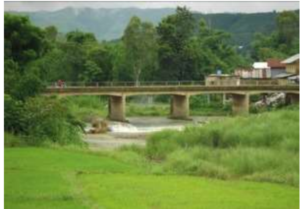
Existing bridge in Pallel
