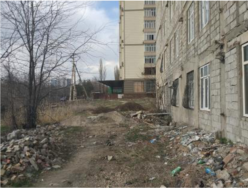
Wastes near the constructing buildings
