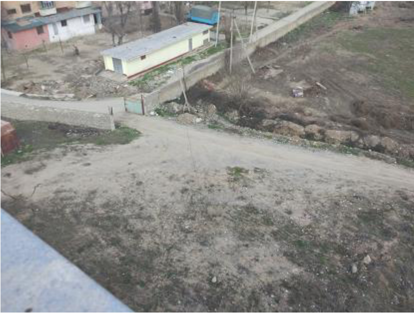
Access road to the campus used for transportation of construction materials
