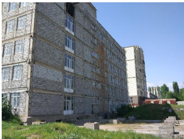
Partially completed Administrative building (Building 1)
