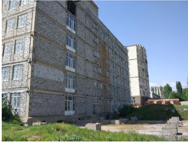
Partially completed Administrative building (Building 1)
