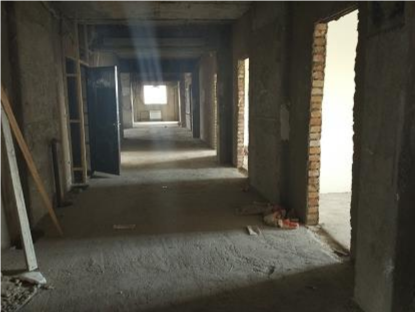
Some premises in process of construction by Hydromet agency (government budget)
