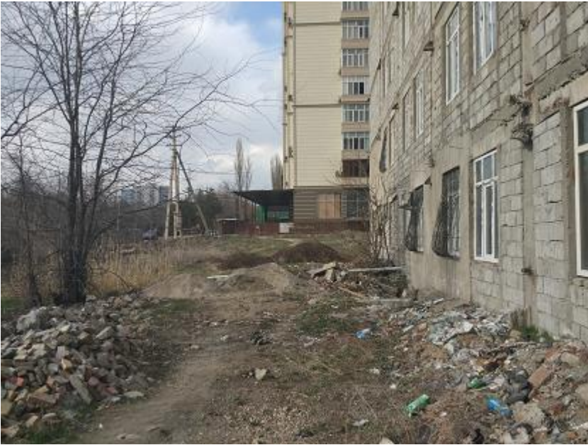
Wastes near the constructing buildings
