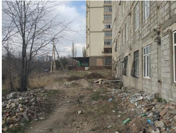
Wastes near the constructing buildings
