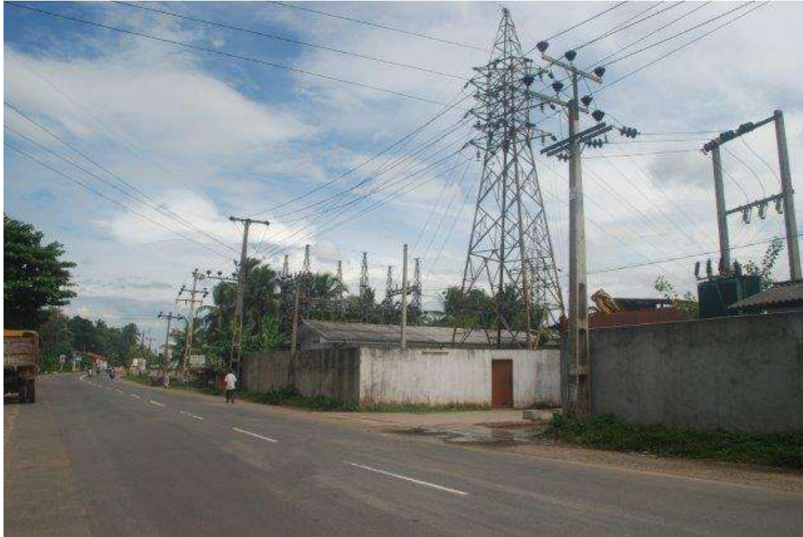
(Existing Ambatale Gantry)
