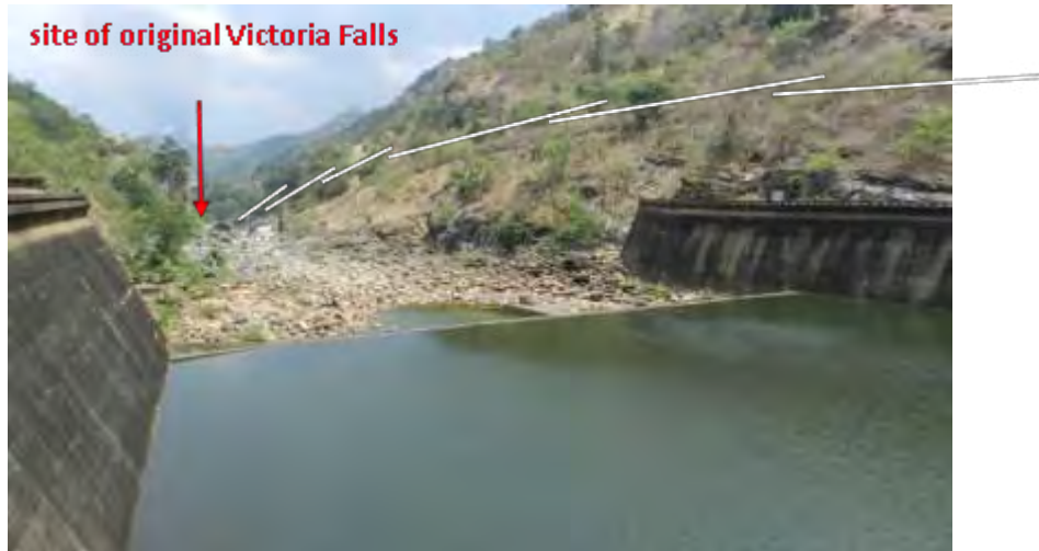
Photo 10: Tailrace at the Victoria Dam (slope trending lines have been inserted).
