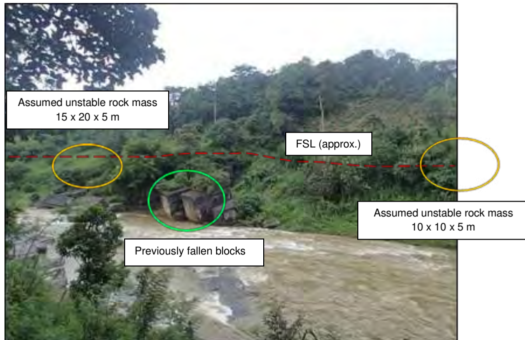
Photo 8: Unstable rock masses on right bank 1 km upstream of dam site
