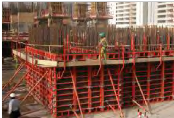
Photo 6: A typical picture of a steel and plywood formwork
