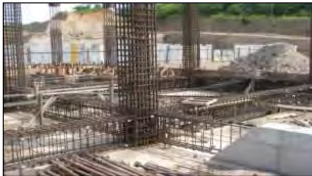
Photo 5: A typical picture of a steel reinforcing for building foundations and small structural columns
