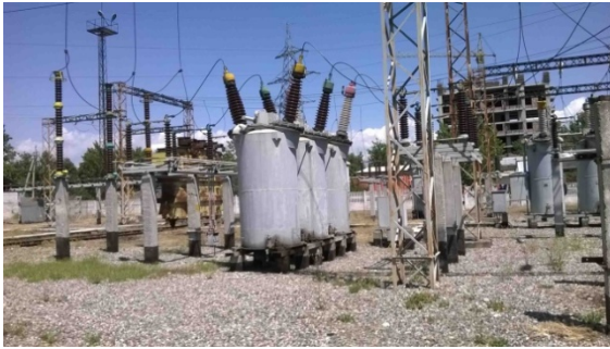
Figure 3-12 Oil filled circuit breaker with two CT's
