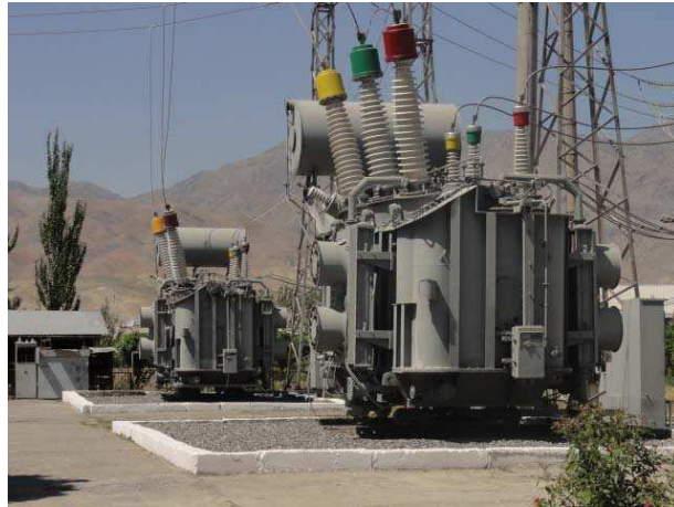
Transformer at s/s Rudaki to be exchanged
