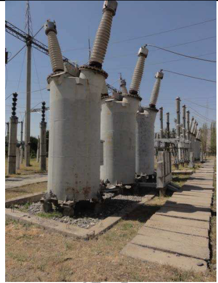
Circuit breakers at s/s Rudaki to be exchanged
