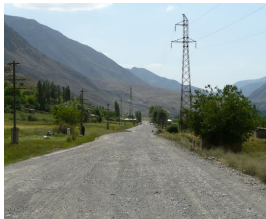
Figure 10-2 old 110 kV line from Ayni to Penjikent. Both examples show towers using non-used land of little value near to roads
