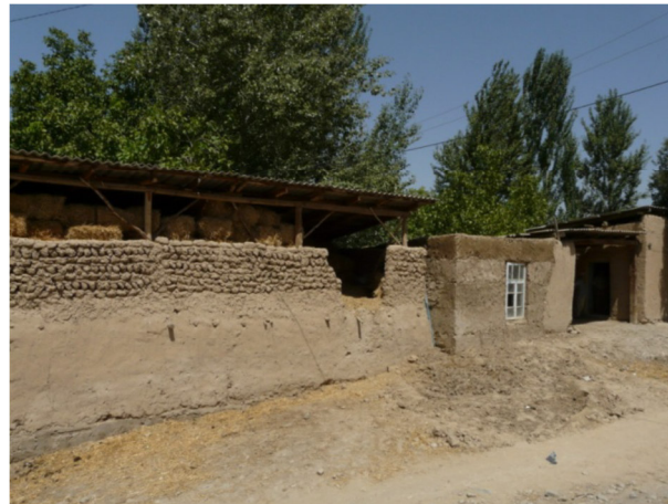
Figure 10 very simple farmstead made by sun dried bricks made of clay
