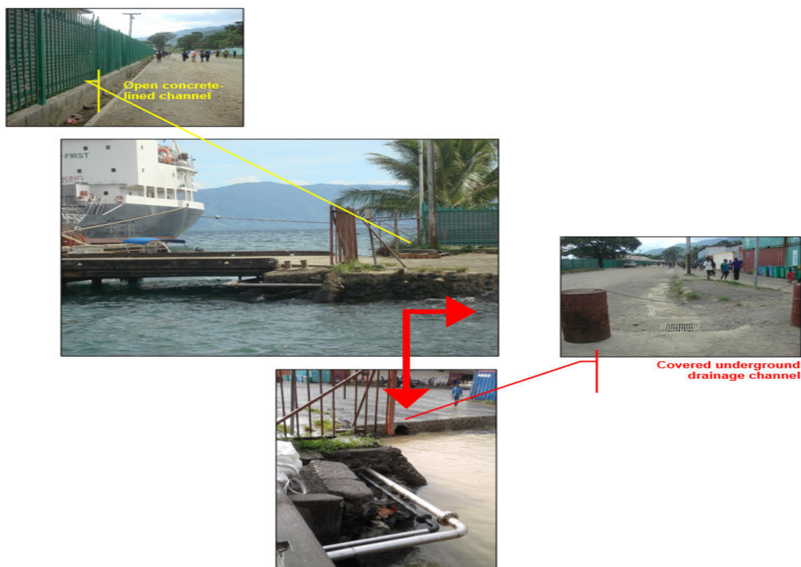
Figure 3.1: Drainage Discharge Points at Seawall and Current Backflow During High Tide Level
