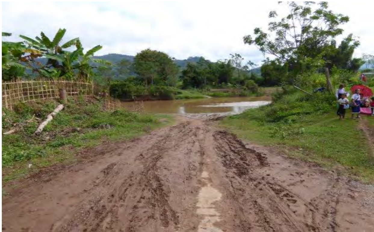
Figure 29. Site of new bridge on Nam Tha river for new road east to Thongdi village
