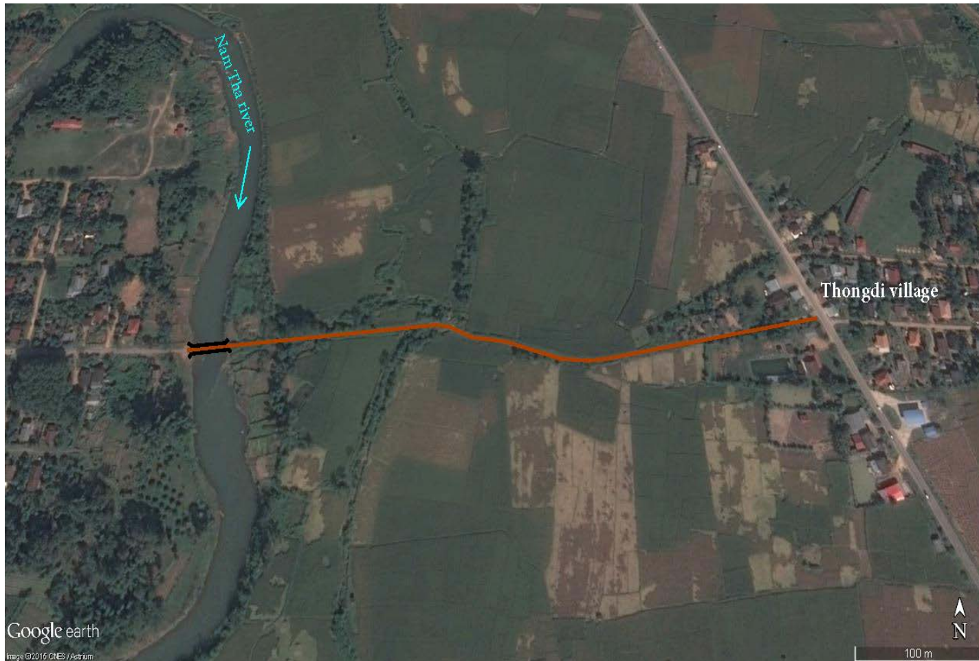
Figure 17. New road and bridge over Nam Tha river
